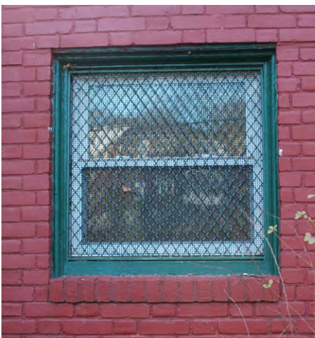
Figure 4: Original wood casing at window opening.
