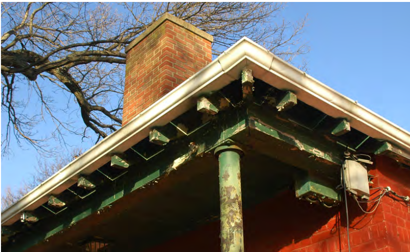
Figure 3: Exposed brackets below hipped roof at rear elevation.
