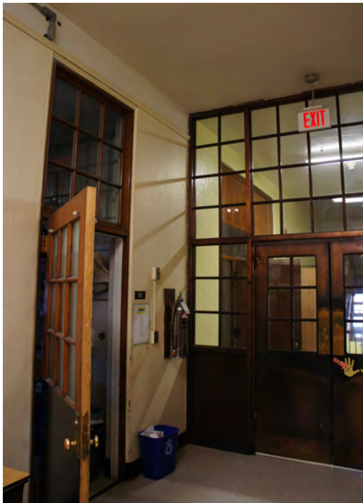
Figure 3: Typical classroom door and stairwell/corridor dividing wall.
