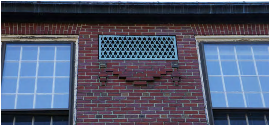
Figure 5: Grille and associated brick swag detail.
