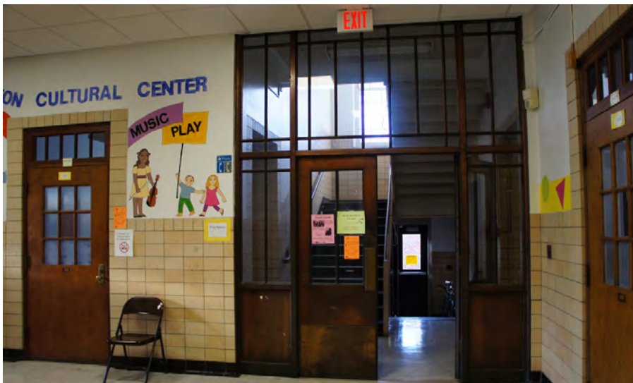
Figure 6: Metal clad partition and doors between first floor corridor and stairwell.
