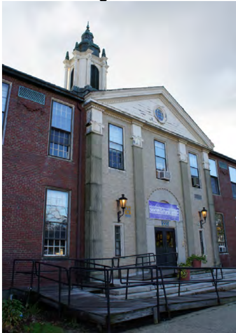
Figure 3: Central entrance bay with its mix of masonry and wood elements.
