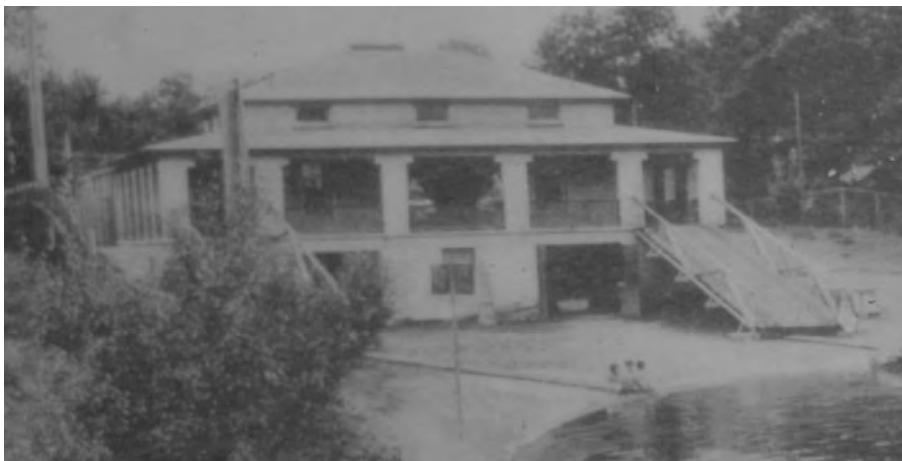
Figure 2: postcard detail. Note the ramps at the north and south porch bays.
