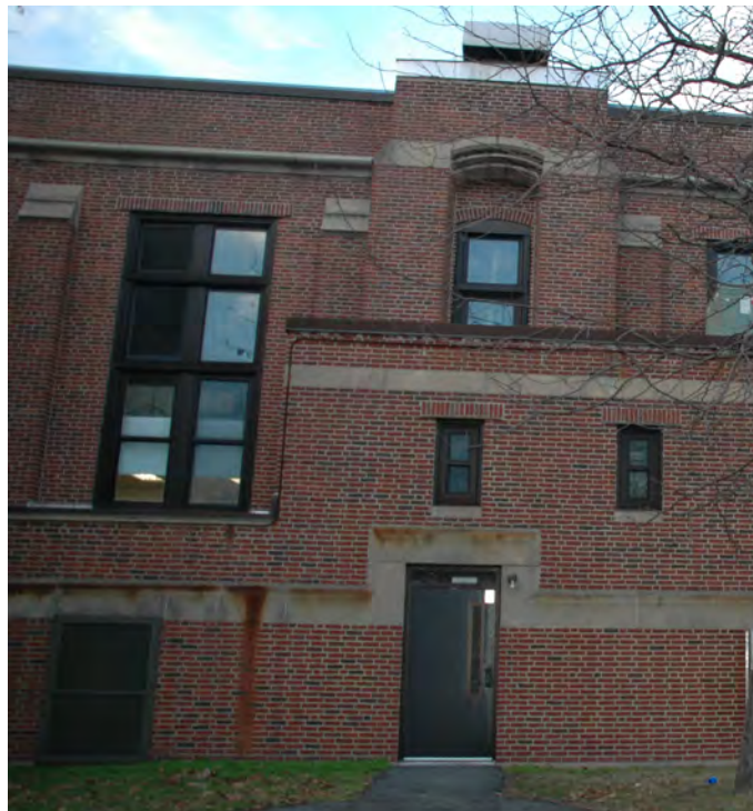
Figure 5: the north (shown) and south sides of the 1934 rear wing are articulated with tall windows between buttresses and a doorway above a lower volume.
