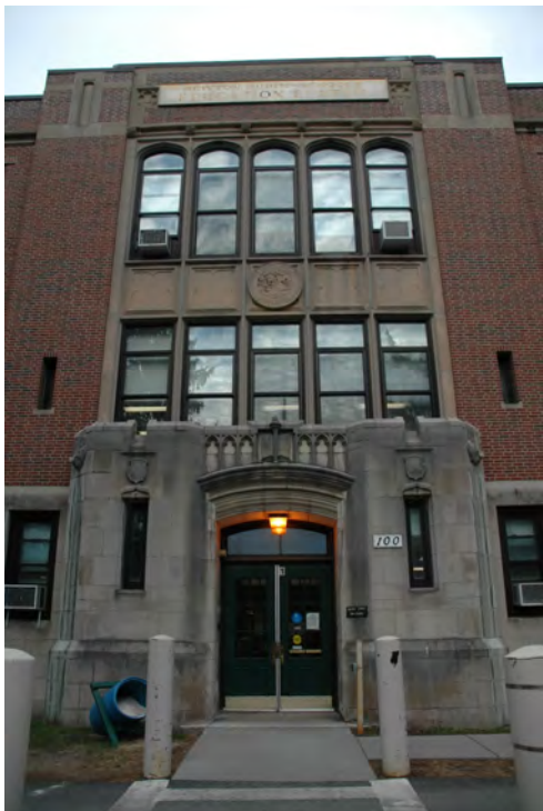
Figure 4: the articulated main entrance bay. Note that the pediment has been removed. Compare with historic photo in Figure 1.
