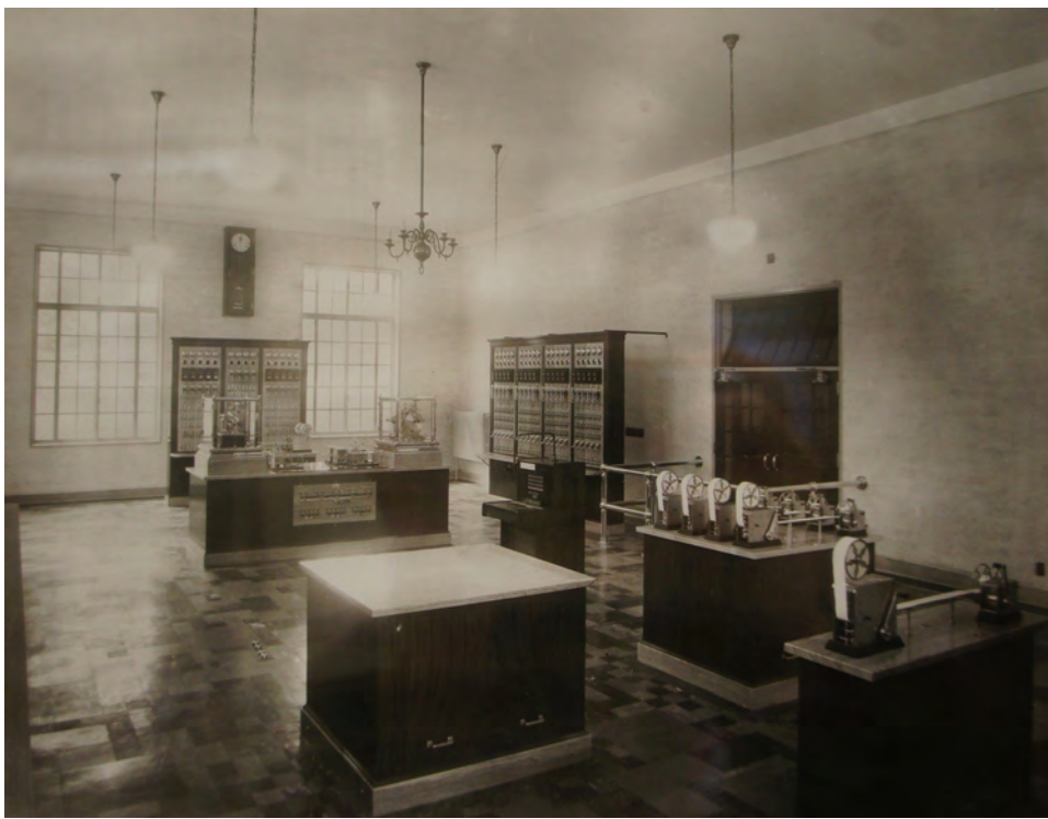
Figure 2: fire alarm equipment, second floor. Note the pair of doors with operable transom and the multi-paned windows. (Credit: Fire Department Headquarters)
