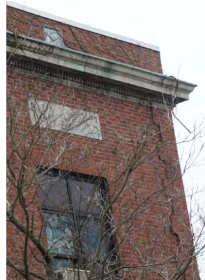
Figure 4: typical window with cast stone panel above. Note the brick quoins at the corner and the small cast stone panel within the parapet.
