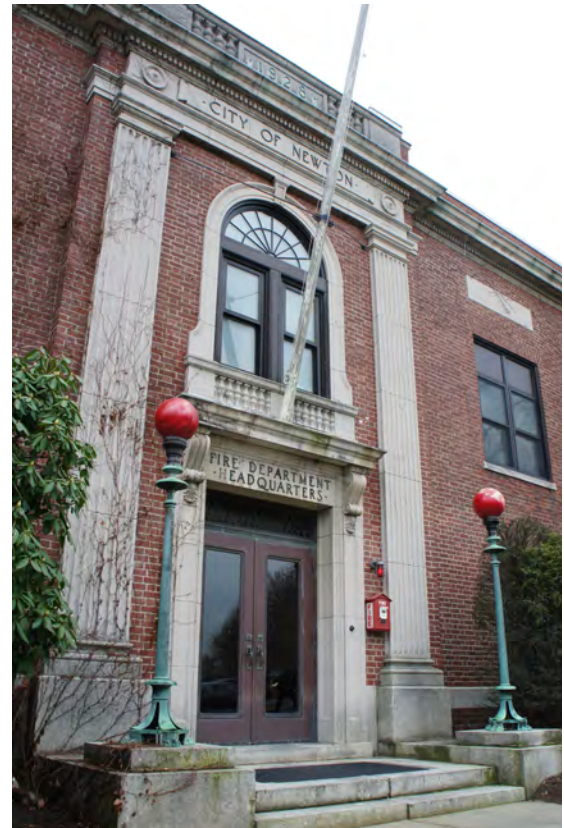
Figure 6: main entrance at west elevation.
