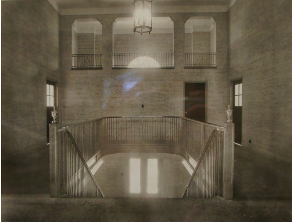
Figure 1: the second floor stair hall (Credit: Fire Department Headquarters)
