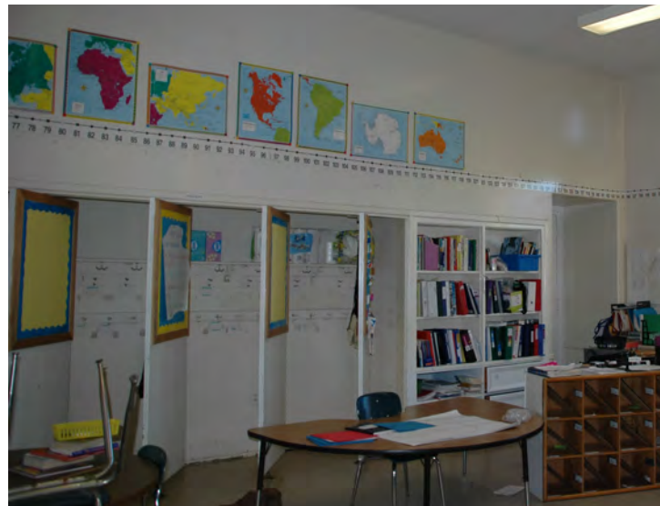
Figure 4: original set of pivot doors at a wide, shallow coat closet, typical in each classroom. The doors have been removed from many classrooms, but in many cases the hardware remains.
