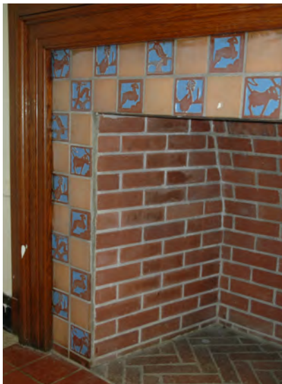
Figure 3: decorative fireplace on the first floor is characterized by the animal print ceramic tiles on the surround.
