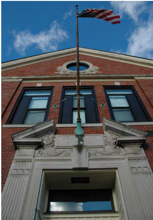
Figure 1: front entry characterized by the door surround, flagpole, and decorative circular window centered within the pediment.
