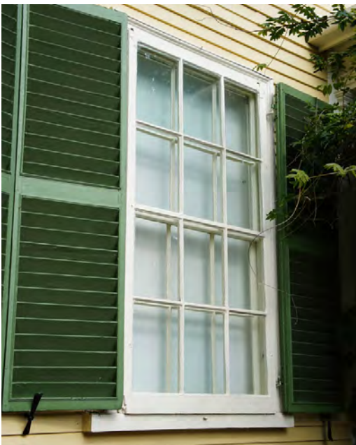
Figure 6: Window with exterior storm.
