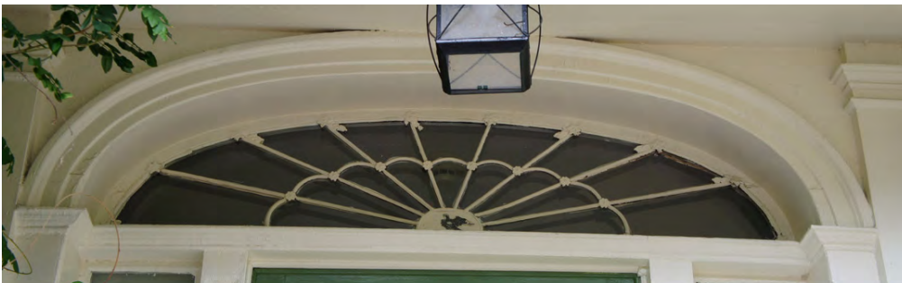
Figure 5: Detail of elliptical fanlight.
