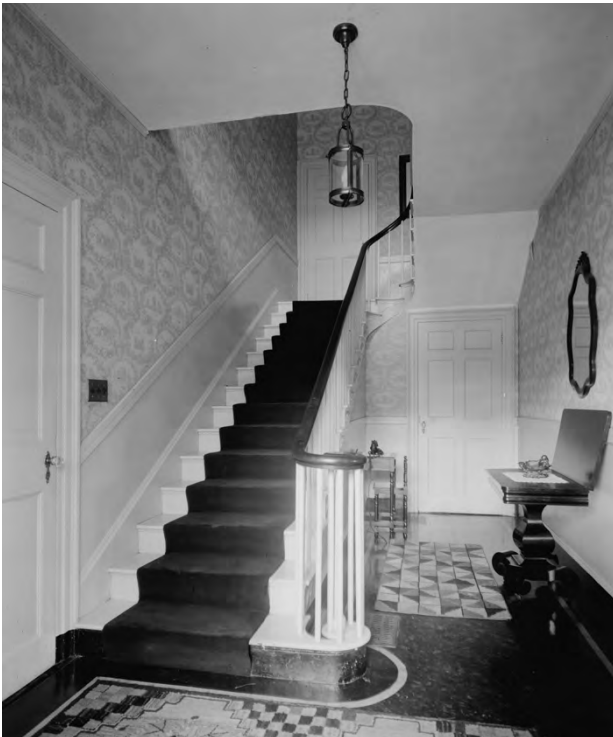
Figure 2: Interior stair-hall in the Jackson Homestead, 1935 (Credit: Library of Congress, Historic American Buildings Survey, Arthur C. Haskell, Photographer).
