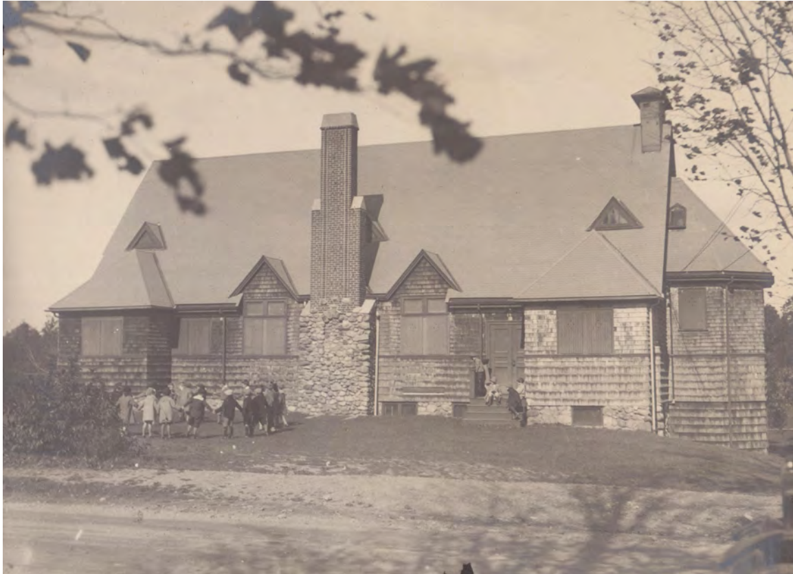
Figure 2: Image from 1925. Note the shingles, which appear to have been unpainted, and the no longer extant dormers. (Credit: Historic Newton)
