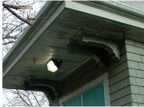
Figure 5: ornamental wood brackets at the west entry vestibule
