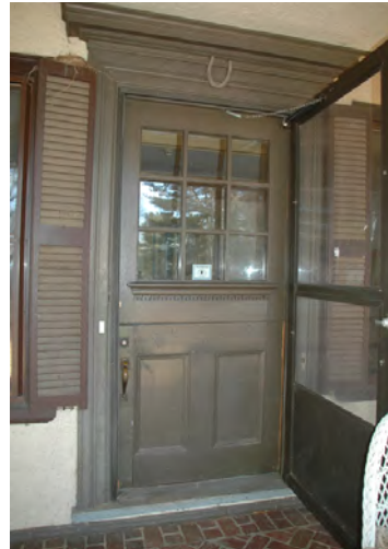
Figure 4: Exterior wood door with original hardware.
