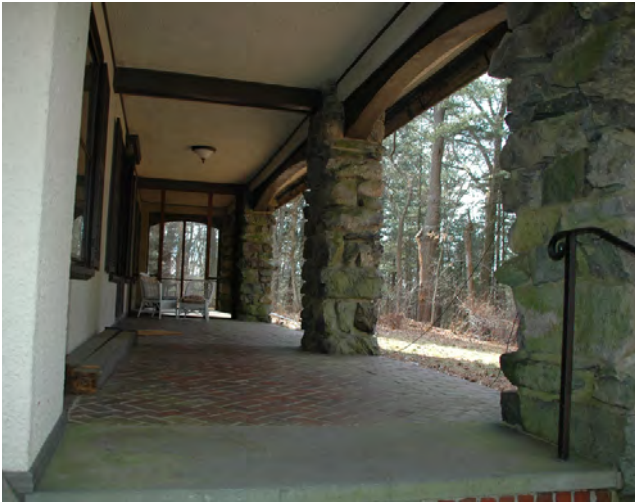
Figure 3: Main exterior porch at west elevation. Note stone columns and wood beams.
