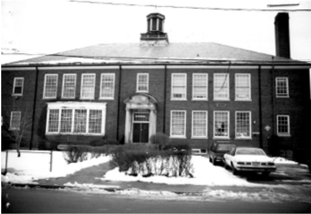
Figure 1: The Lincoln-Eliot School in 1987 prior to the replacement of the original window sashes. (Credit: MACRIS)
