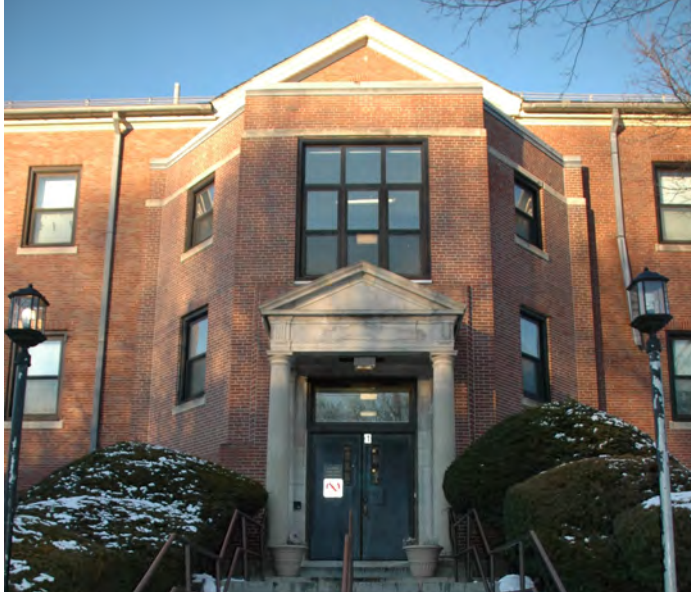
Figure 1 (top left): The current main entry is demarcated by a limestone pedimented portico at the southern, narrow end of the historic building, at the top of a large set of exterior stairs.
