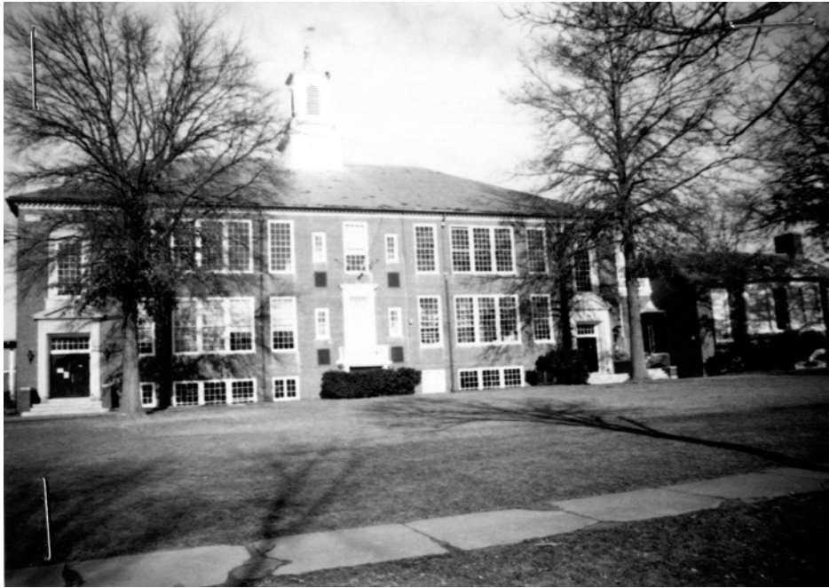
Figure 1: Front elevation of the school circa 1987 (credit: MACRIS).
