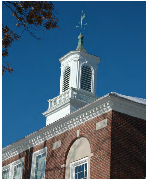
Figure 4: Cupola at main roof.
