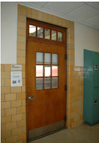
Figure 5: Tile wainscot and door surround in corridor.
