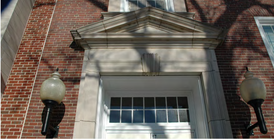
Figure 2: Close up view of stone entrance surround and door transom at main building.
