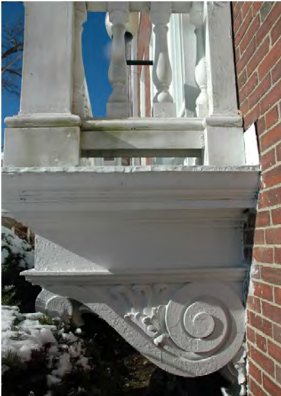
Figure 3: Decorative wood bracket below projecting balcony at south elevation.
