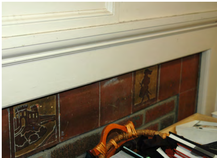
Figure 6: Decorative tilework at fireplace surround of former library space.
