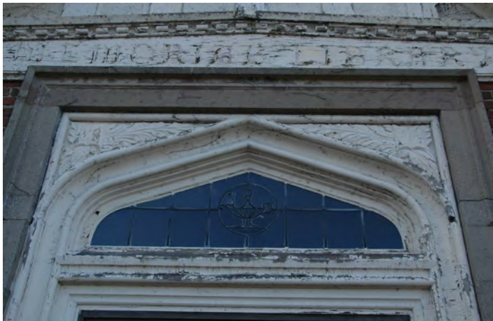
Figure 4: "Memorial Library" carved into the wood above the front door. Note also the oil lamp image in the leaded glass transom.
