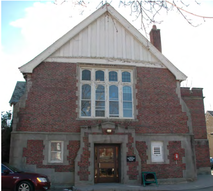
Figure 3: the north gable end exhibits many character-defining features. Note the roofline with the subtle splay at the eaves; the wood and stucco pediment; the large set of leaded glass wood windows set within a cast stone surround; the buttresses shaping the north and south profile of the building; the projecting basement entryway.
