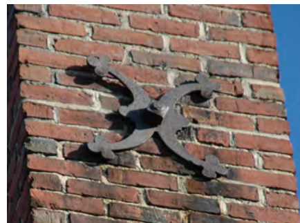
Figure 6 (below): ornamental wrought iron chimney wall tie
