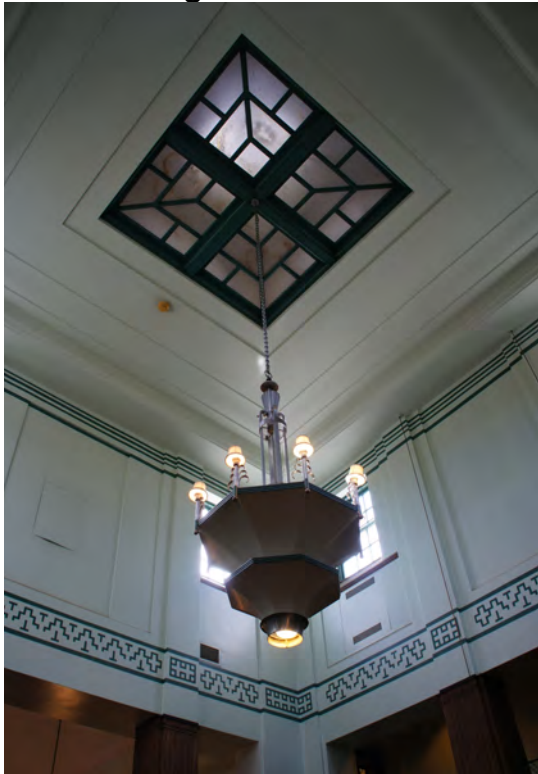
Figure 2: Laylight and chandelier in Main Lobby. Note stepped plaster detail at walls and ceiling.
