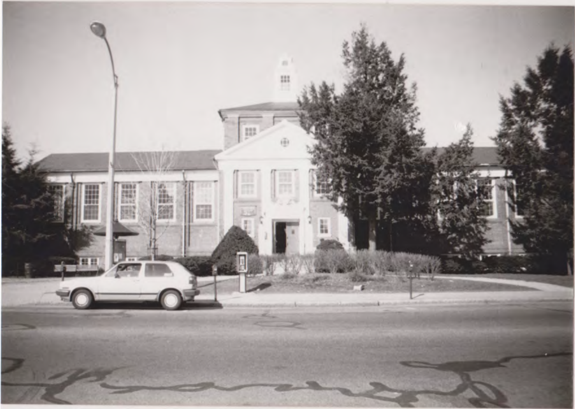
Figure 1: East elevation of Newtonville Branch Library, 1987. The landscaping of the site has changed considerably since then. The light fixtures on the limestone standards have also been changed. (Credit: Historic Newton)
