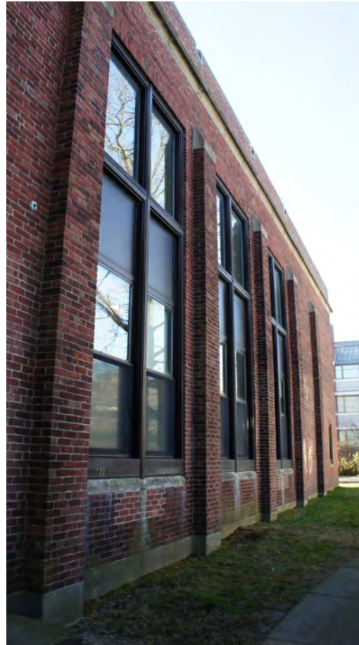
Figure 3: the gymnasium wing is characterized by the tall windows between buttresses; the three cast stone arched doorways on the west façade (not shown) and the round arched arcade to the south, seen below.
