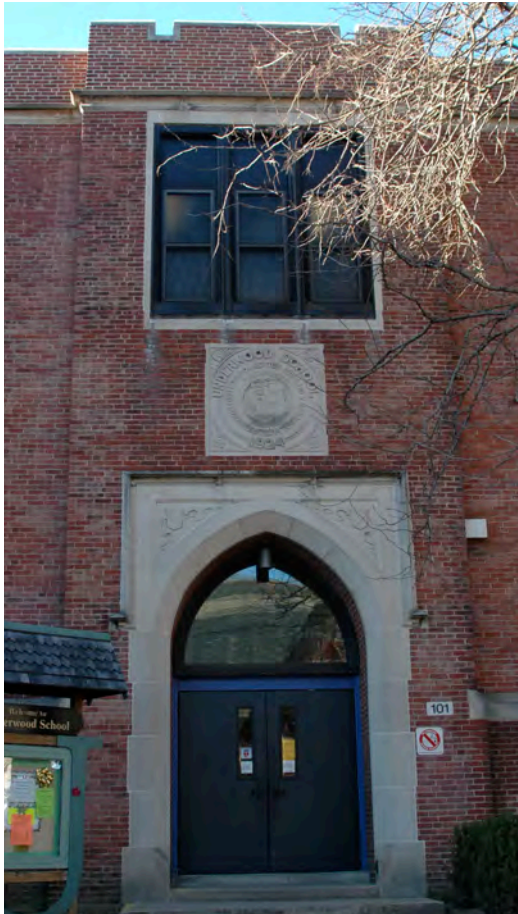
Figure 2: the front entrance on the east elevation (shown), is mirrored with slightly less elaborate secondary entrances to the west and north. Note the crenelated parapet, the cast stone school seal, the elaborate cast stone door surround, and the large windows
