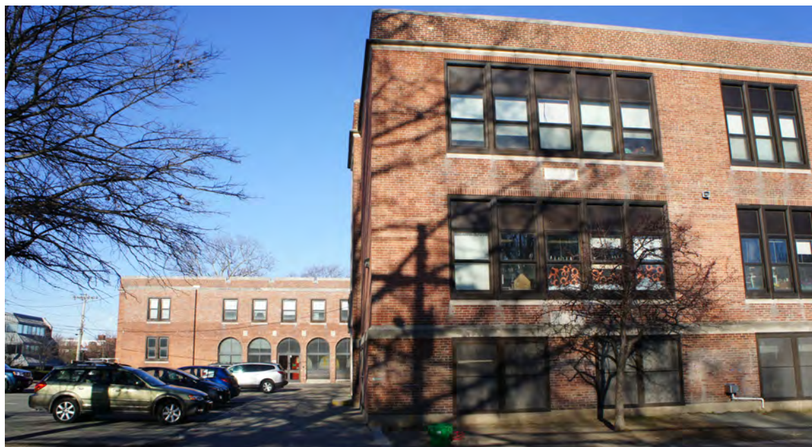
Figure 4: the general rhythm of the building facades is characterized by the large banks of windows seen here in the foreground. The replacement windows drastically affected the character of the building; compare with the historic photo in Figure 1.
