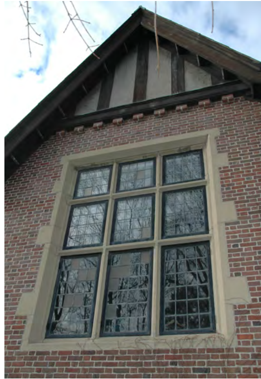
Figure 5: Rear gable- half-timbered detail at top with brick dentils, typical gable-end window.
