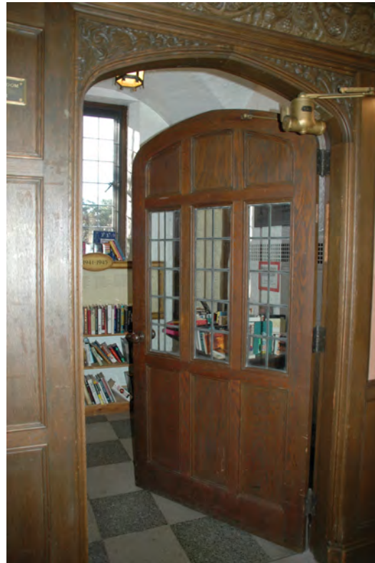
Figure 7: wood paneled door from center hall to the entry vestibule. Lead-camed lights at three panels, arched doorway in wood paneled screen wall with elaborate carvings.
