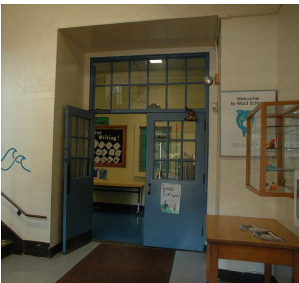
Figure 5: Interior wall partition.
