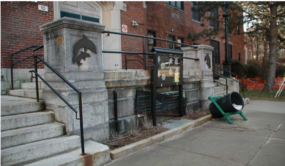
Figure 4: Main entrance staircase.
