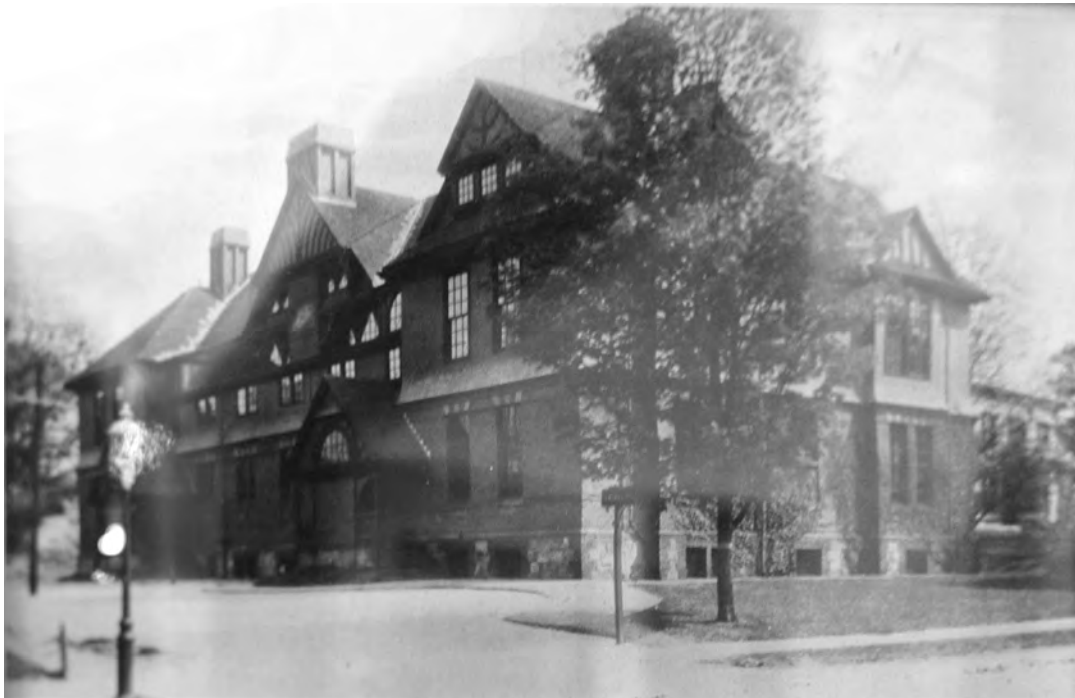
Figure 2: Previous Thomas S. Williams School on Hancock Street, replaced by the current school building. (Credit: Auburndale Library)
