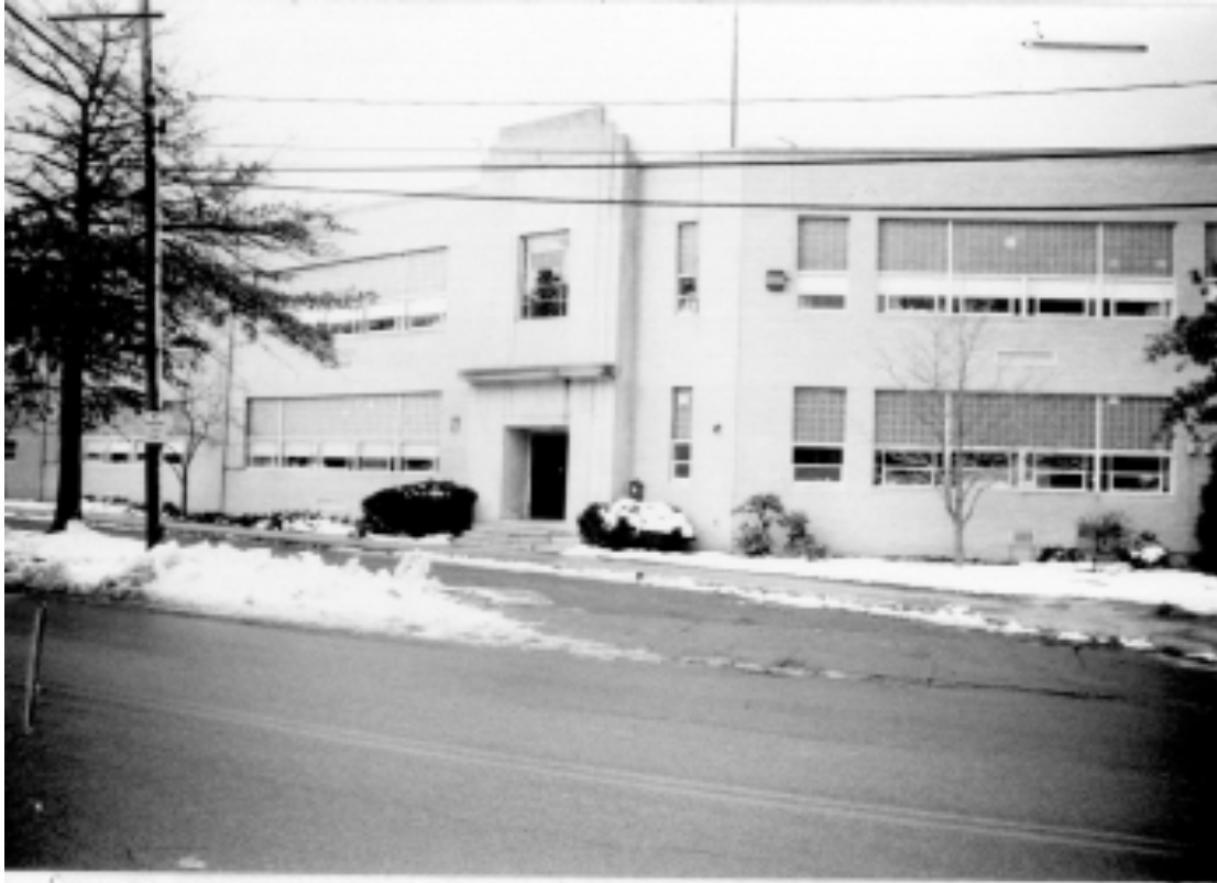
Figure 1: Williams Elementary School circa 1987 showing the original glass block and steel strip windows. (Credit: MACRIS)
