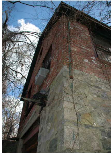
Figure 4: Close up view of the fieldstone foundation.
