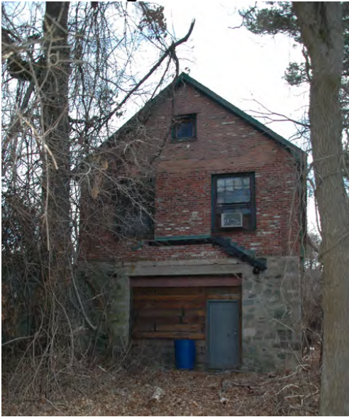
Figure 3: North elevation of garage. Note the remnants of the projecting roof above the opening.
