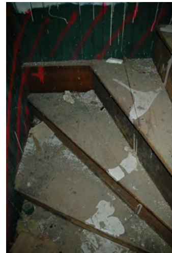
Figure 7: Stairway to the attic with beadboard walls.
