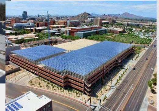
884 kW, Arizona Garage
