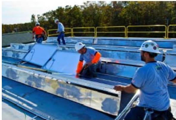
Panel Assembly & Wiring
