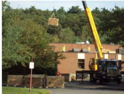
Mobilization & Crane Ops
