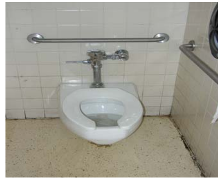
Flushometer (tankless) toilets will be retrofitted.
