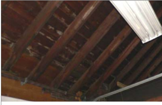
Thermal Panel Installation (Attic)
