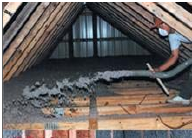
Cellulose Installation
