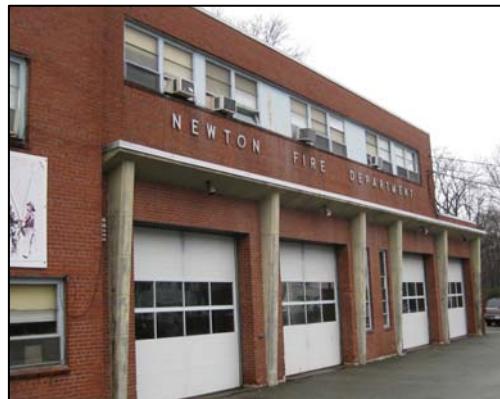
Fire Station 3 Apparatus Bays
