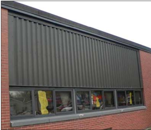
Thermal Panel Installation (Windows)
