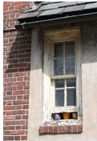
Existing Windows at Health Department Headquarters
