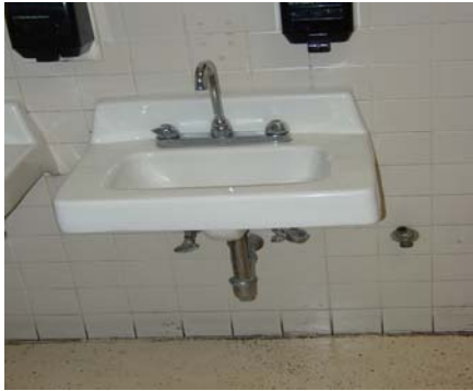
Standard flow aerators will be retrofitted.
