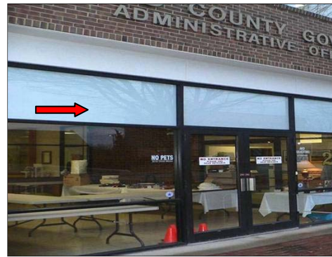
Thermal Panel Installation (Window)
