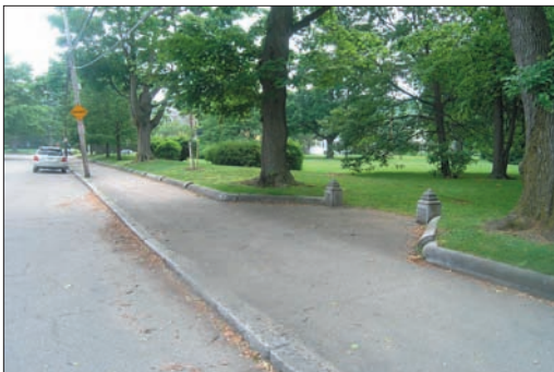
Missing walkway at the historic entrance on Eldridge Street
