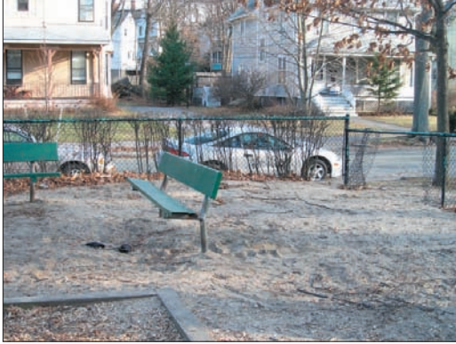
Chain link fence in disrepair
