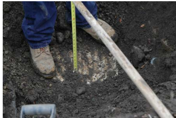
Area 5: intact concrete pool basin 24” below existing grade
