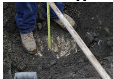
Area 1 second excavation depth of 24” with concrete basin visible
