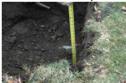
Area 1 initial excavation depth of 18”
