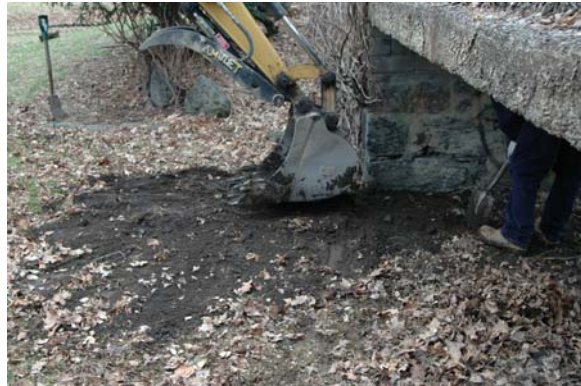
Area 2 excavation location
