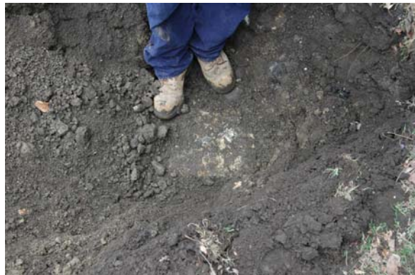
Area 3: intact concrete pond basin, 24” below existing grade
