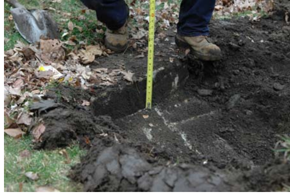
Area 4: 6" vertical reveal of pond edge / coping
