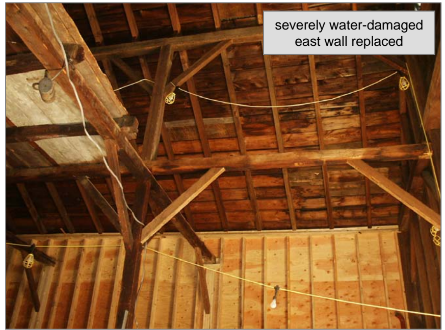
original interior framing preserved & visible
