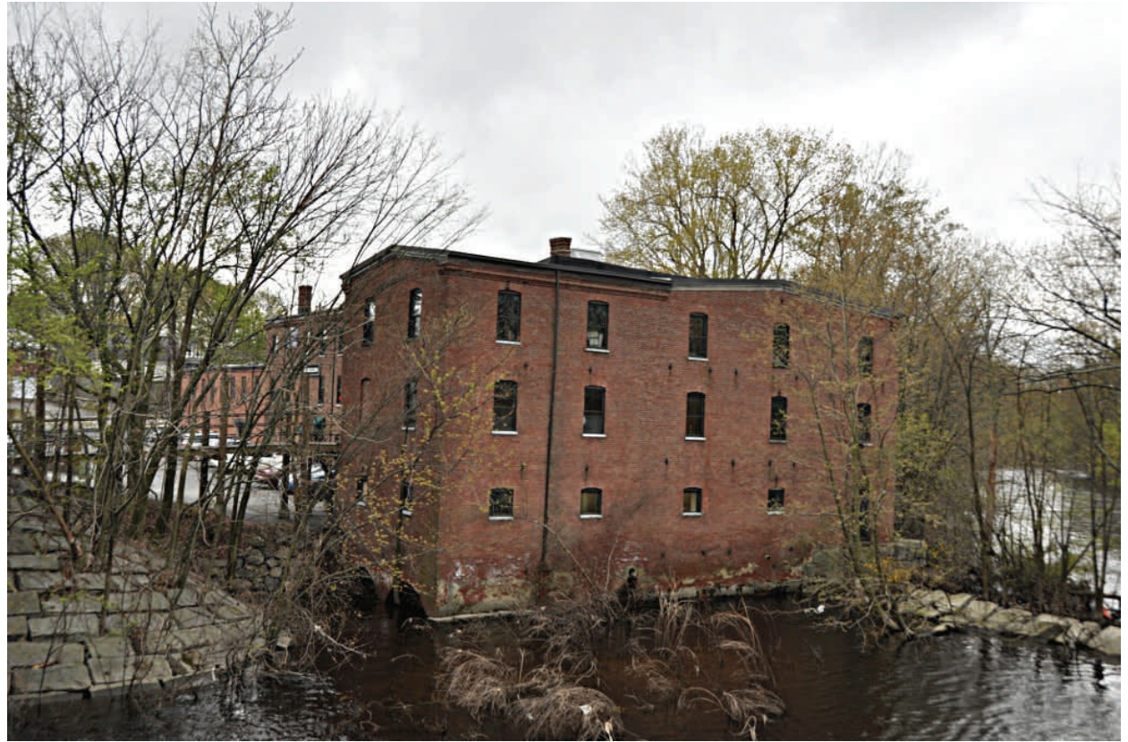
The 1845 Bemis Mill is a historic manufacturing building in the village of Nonantum. ( http://en.wikipedia.org/wiki/File:NewtonMA_BemisMill.jpg )
