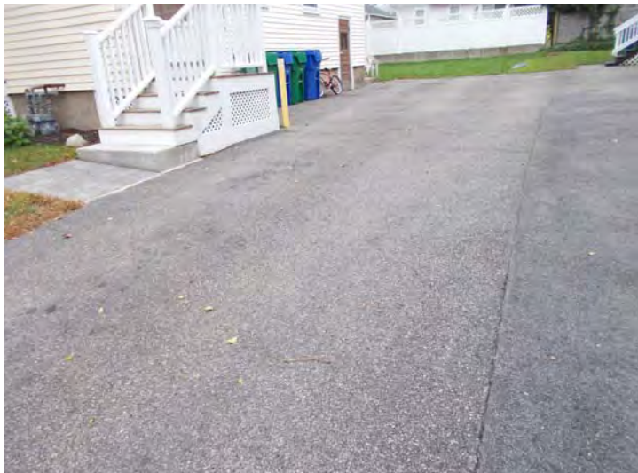
10-12 Cambria Road Driveway
