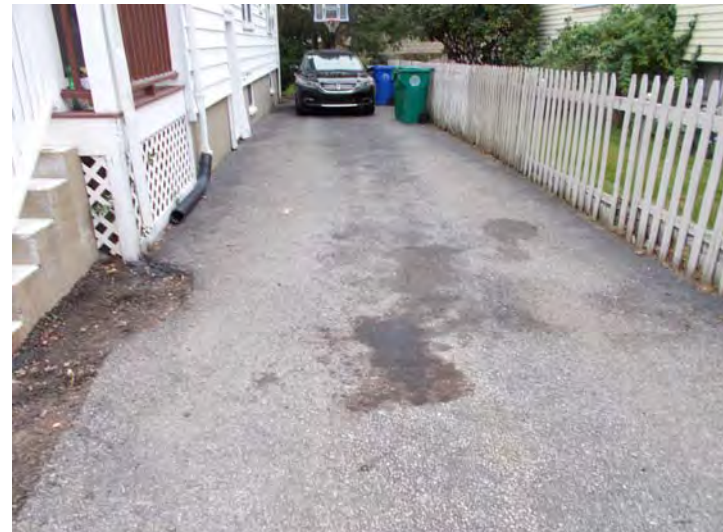
11-13 Cambria Road View of driveway and wood fencing
