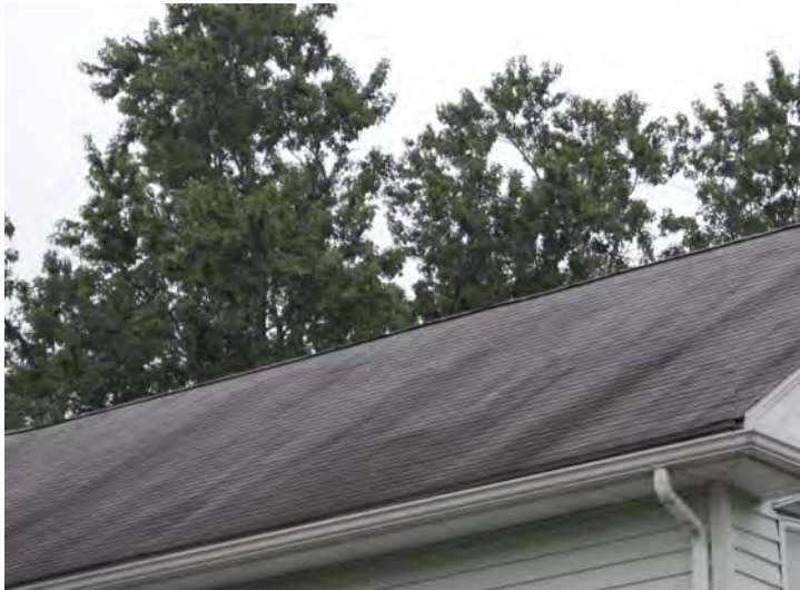
20-22 Falmouth Road View of older asphalt roofing
