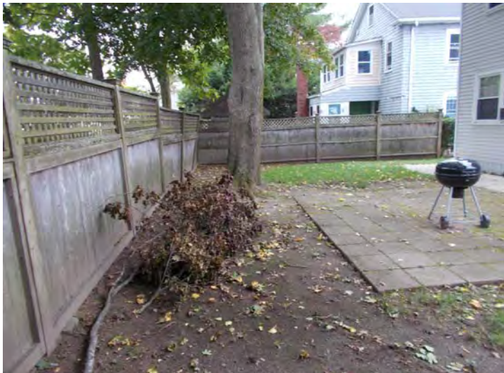
18-20 Cambria Road Wood stockade perimeter fencing
