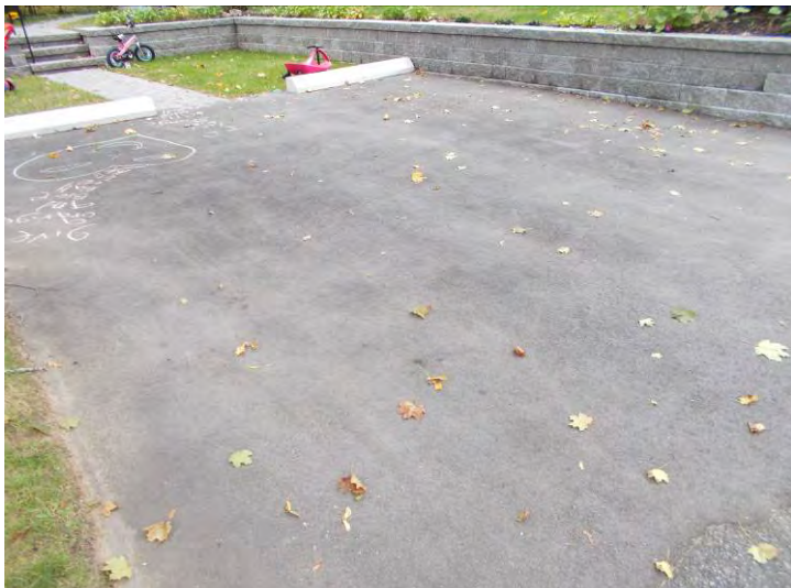
54 Taft Avenue View of parking area
