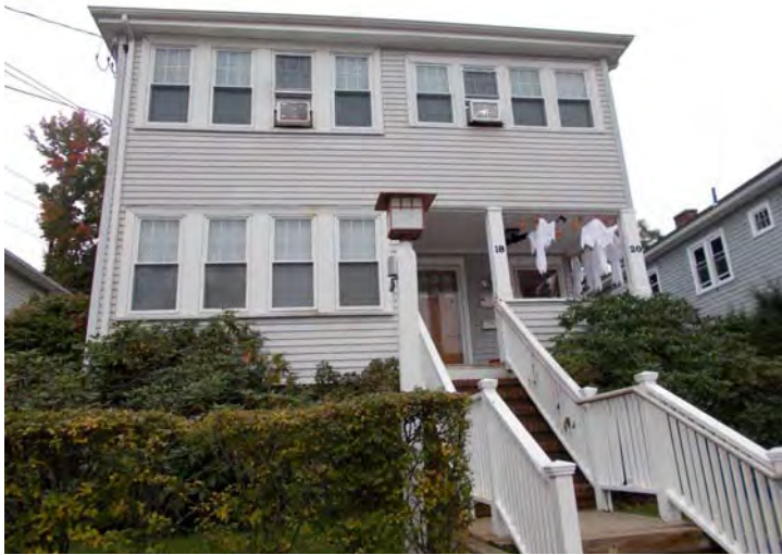
18-20 Cambria Road Front façade
