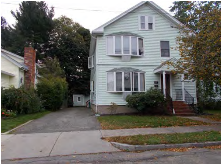
20-22 Falmouth Road View of front façade and driveway
