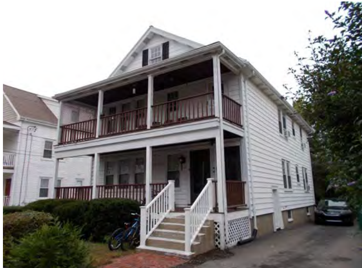
11-13 Cambria Road Front façade
