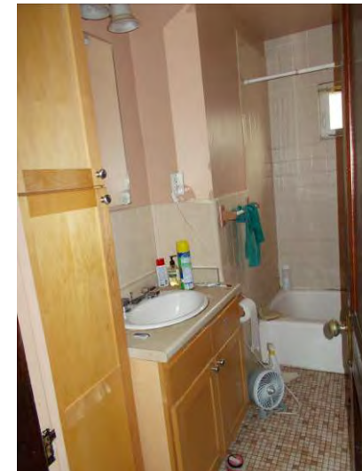
163 Jackson Road View of second floor bathroom
