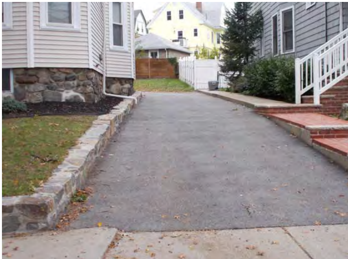
54 Eddy Street View of asphalt driveway
