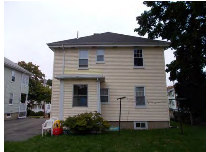
10-12 Cambria Road Rear facade
