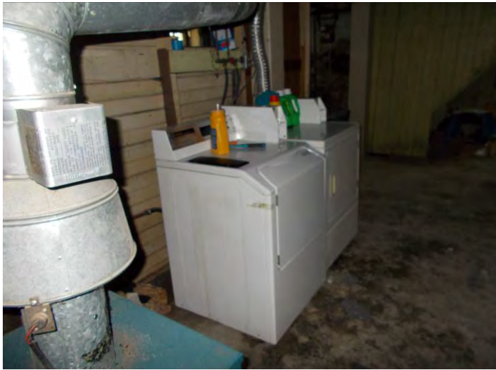
163 Jackson Road Basement level laundry room
