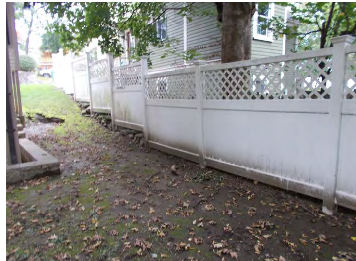
14 Nonantum Place Vinyl fencing at site perimeter
