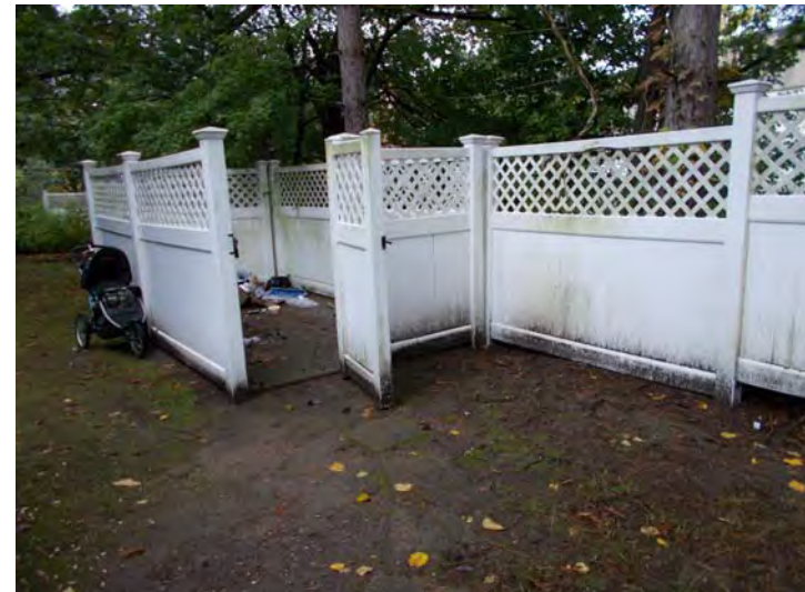
90 Christina Street Vinyl stockade fencing at site perimeter
