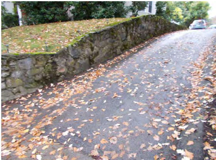
2148-2150 Commonwealth Avenue Driveway and stone retaining wall
