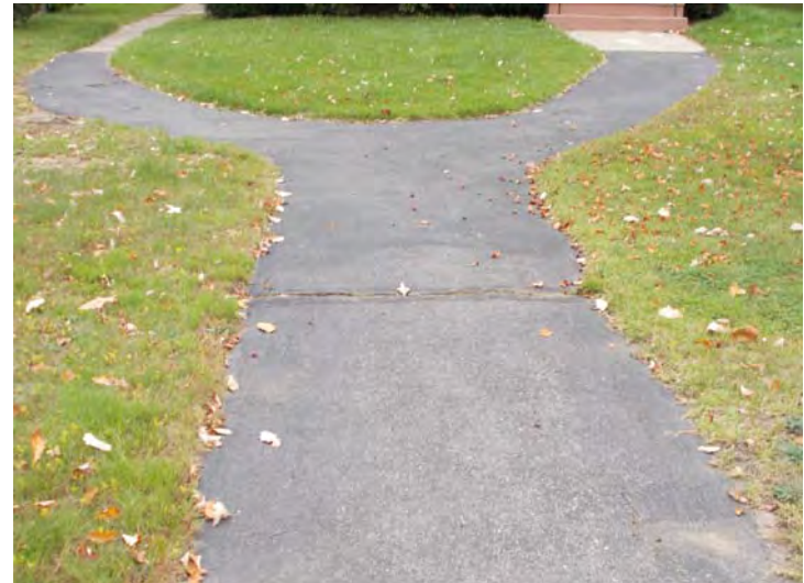
163 Jackson Road Front asphalt walkway
