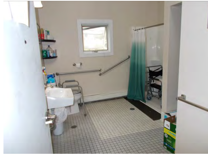
228 Webster Street View of first floor accessible bathroom
