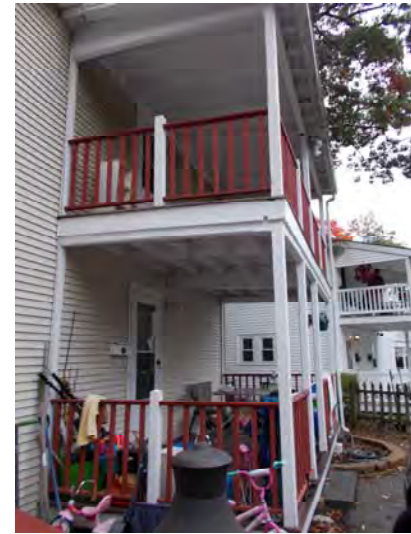
2148-2150 Commonwealth Avenue Rear back decks replaced in 2010
