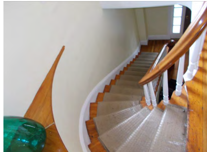
61 Pearl Street View of common stairway
