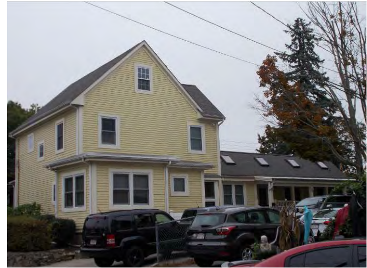
228 Webster Street Rear and side façade
