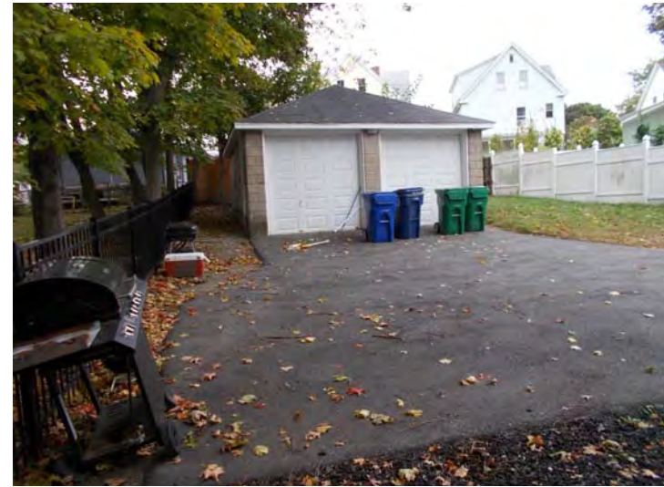
54 Eddy Street Garage and rear parking area
