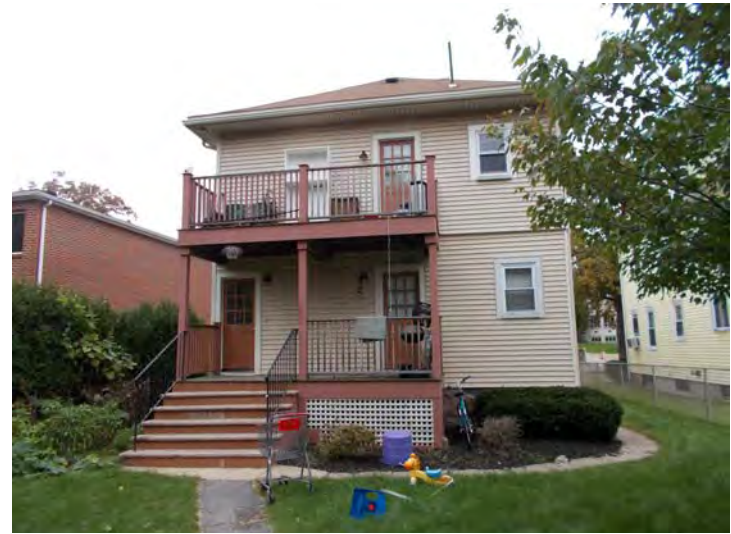
163 Jackson Road Rear facade
