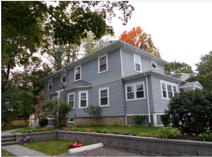
54 Taft Avenue Front façade
