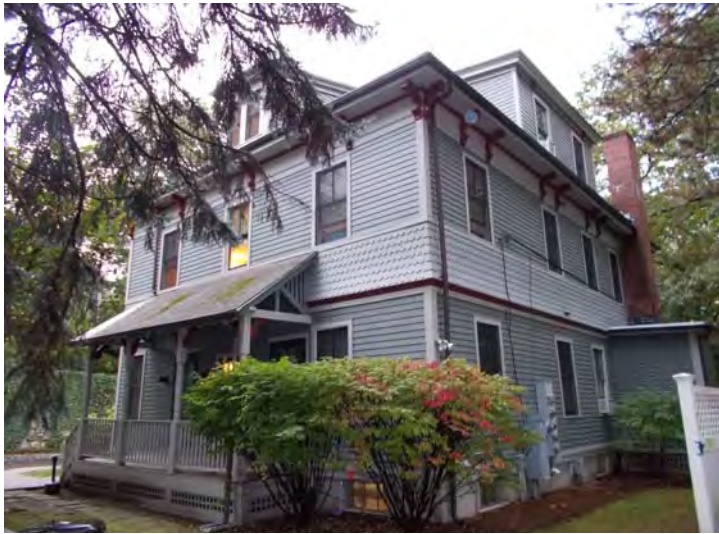
90 Christina Street Rear and side façade; note recently painted
