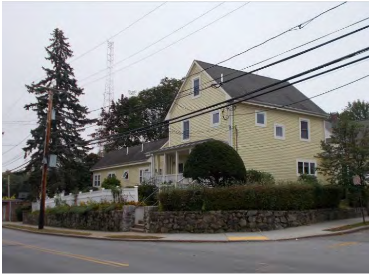
228 Webster Street Front façade
