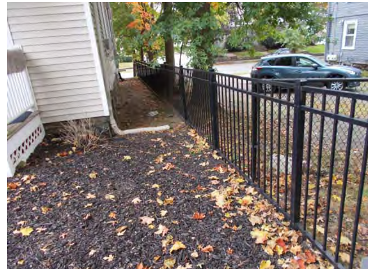
54 Eddy Street Metal rail fencing at side property line
