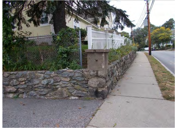
228 Webster Street Stone retaining wall
