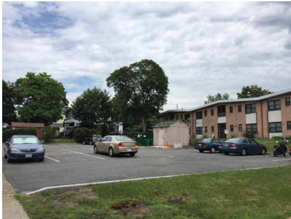
Existing Parking Lot
