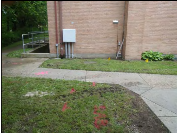
Photo 1 View of the Site looking in a southwesterly direction towards Building 105 on May 26, 2017.
