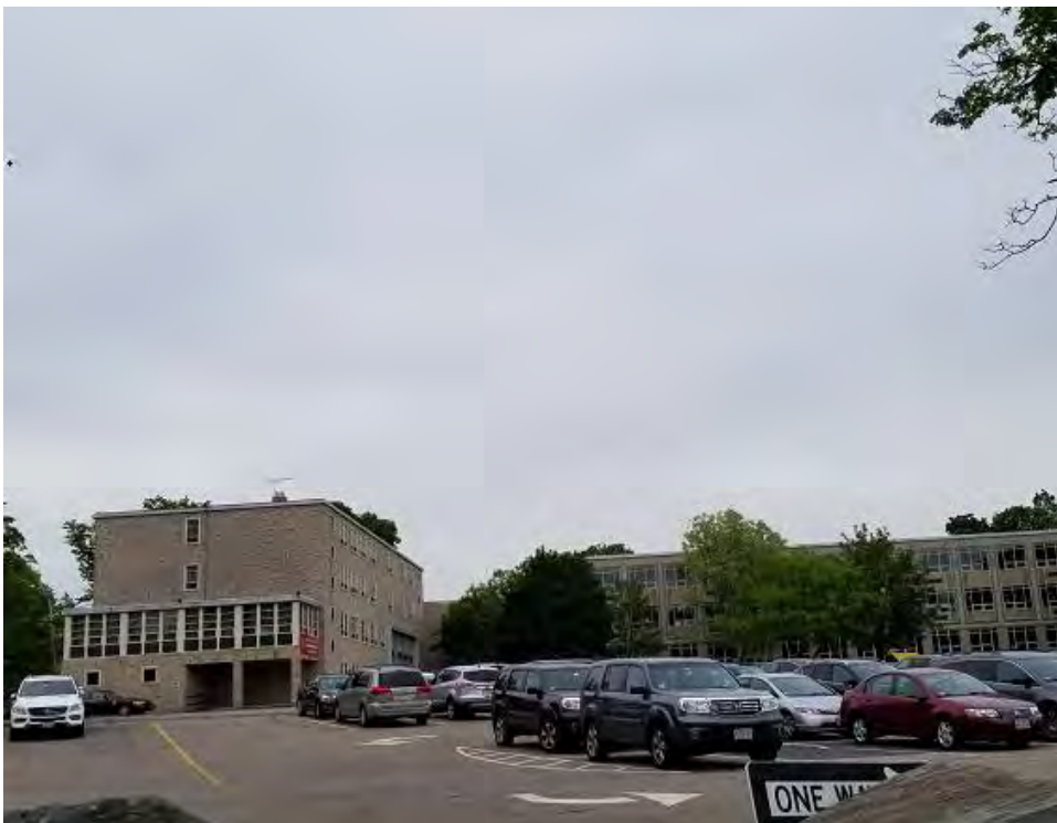
View of the Jackson private elementary school located across from the subject site
