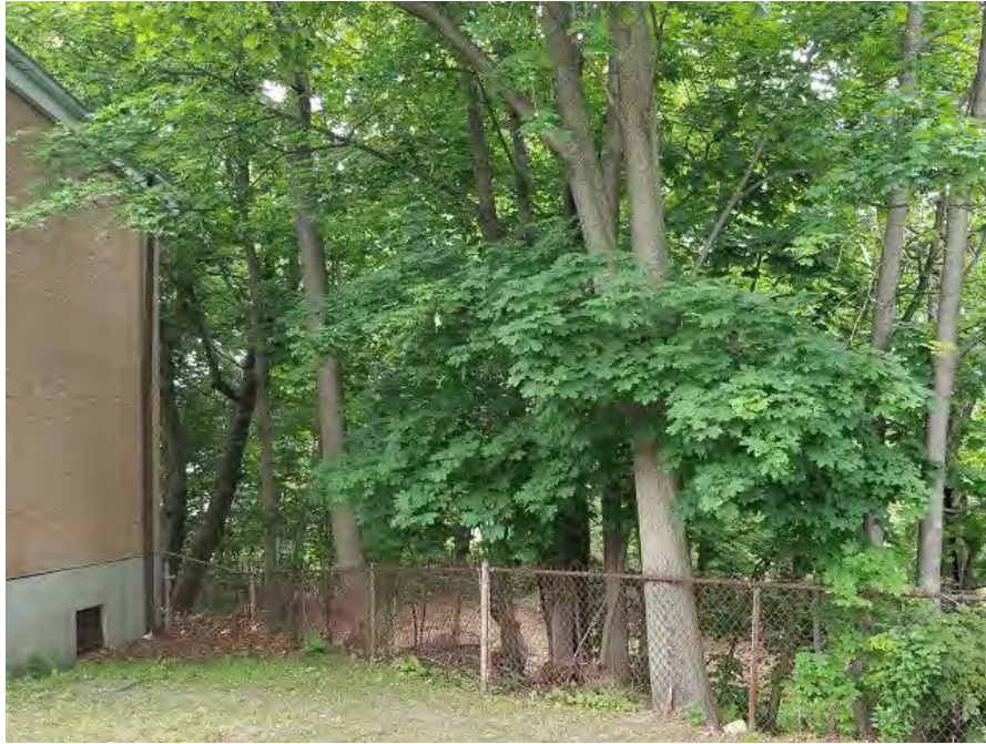
View of the subject site from the Jackson Gardens development
