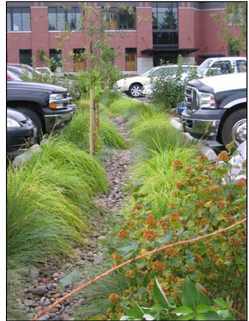
Parking lot runoff is allowed to infiltrate through a vegetated bioretention area
