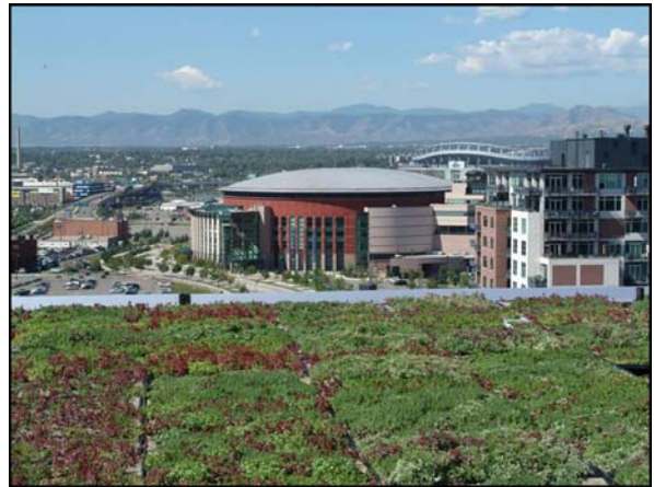
Green roofs capture rainfall, promote evapotranspiration, and offer energy savings. This is a photo of a green roof on the EPA Region 8 building in Denver, CO.
