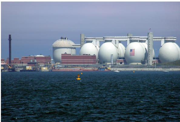
Deer Island Wastewater Treatment Plant
