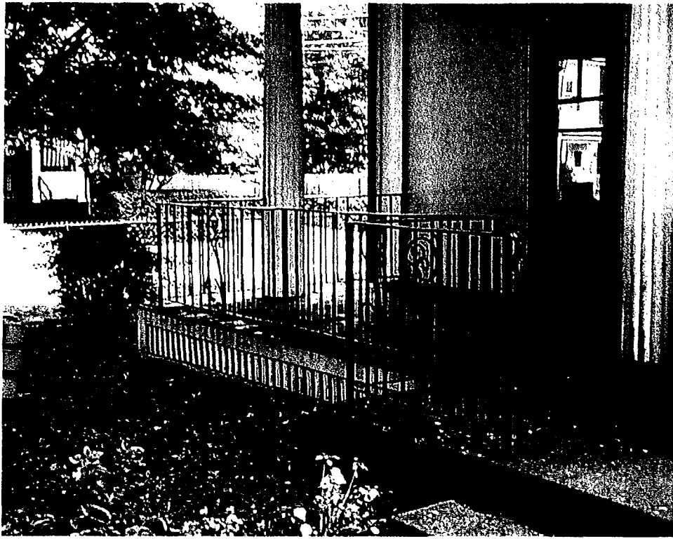
Wrought Iron Railings To Be Removed
