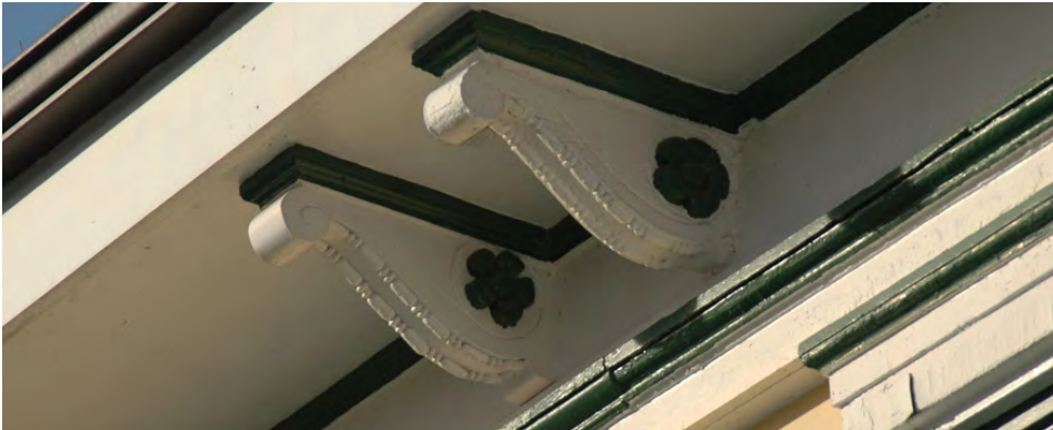
Figure 5: Eave brackets at main building roof.
