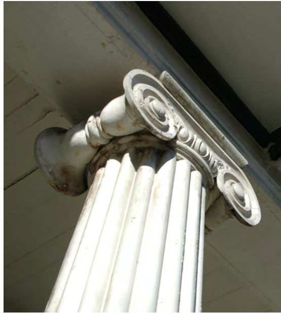
Figure 4: Close up view of ionic column capital at east porch.
