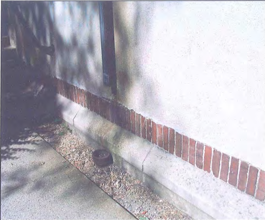
Missing Downspout
