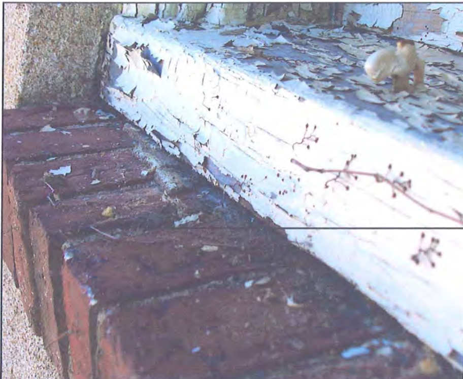
Detail of Brick Window Sill-
