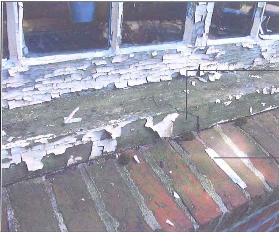
Window Type B1 - North Elevation- Sill Rot
