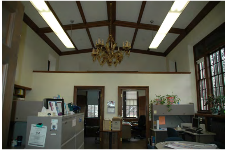
Figure 2: the former west reading room has been subdivided into offices at the west end.
