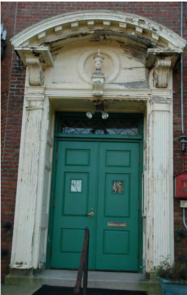
Figure 3: the main entry doorway, with a pair of wood paneled doors and ornamental leaded glass transom within a detailed wood architrave. x
