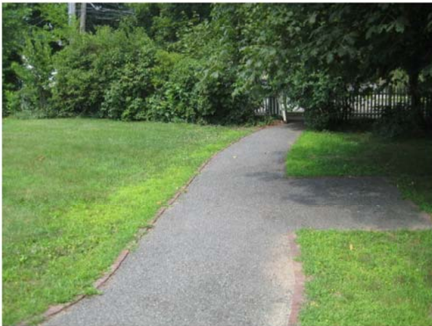
15. Bituminous Sidewalk at Rear of Property
