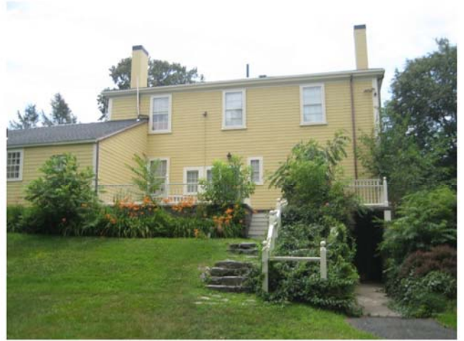
4. Rear Elevation of Historic House
