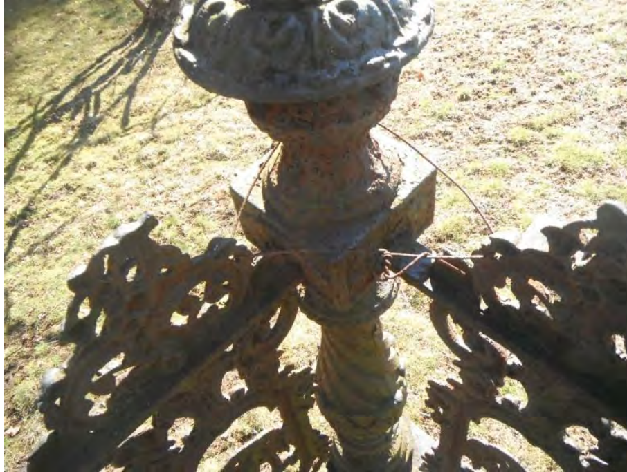
Detail: Wire holding posts to medallions.
