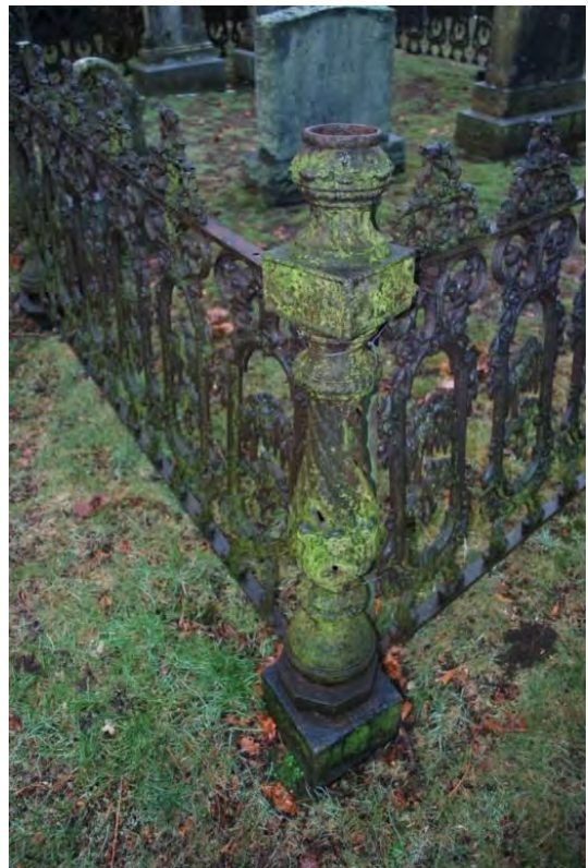
The fence was originally painted black, and the majority of it has deteriorated. The fence is dirty and green biological growth is visible.
