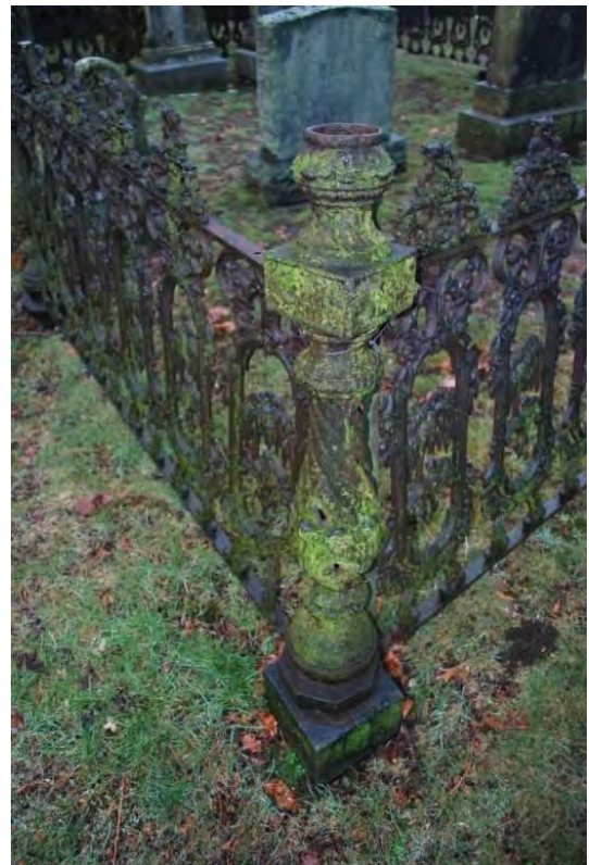
The fence was originally painted black, and the majority of it has deteriorated. The fence is dirty and green biological growth is visible.
