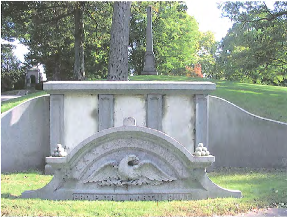
Photo A – Central Portion of Retaining Wall with Obelisk in Background and Cartouche from Top of Monument on Ground in Front of Monument
