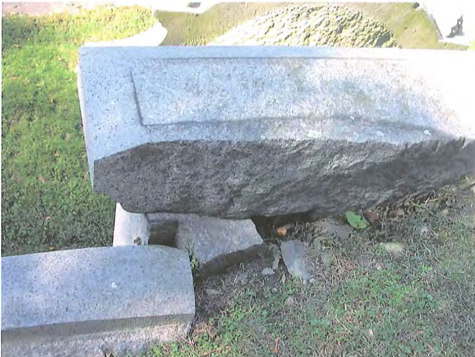
Photo F - Gaps Left by Differential Movement of Various Pieces of the Monument
