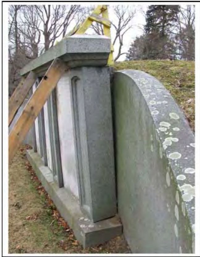
Temporary bracing
