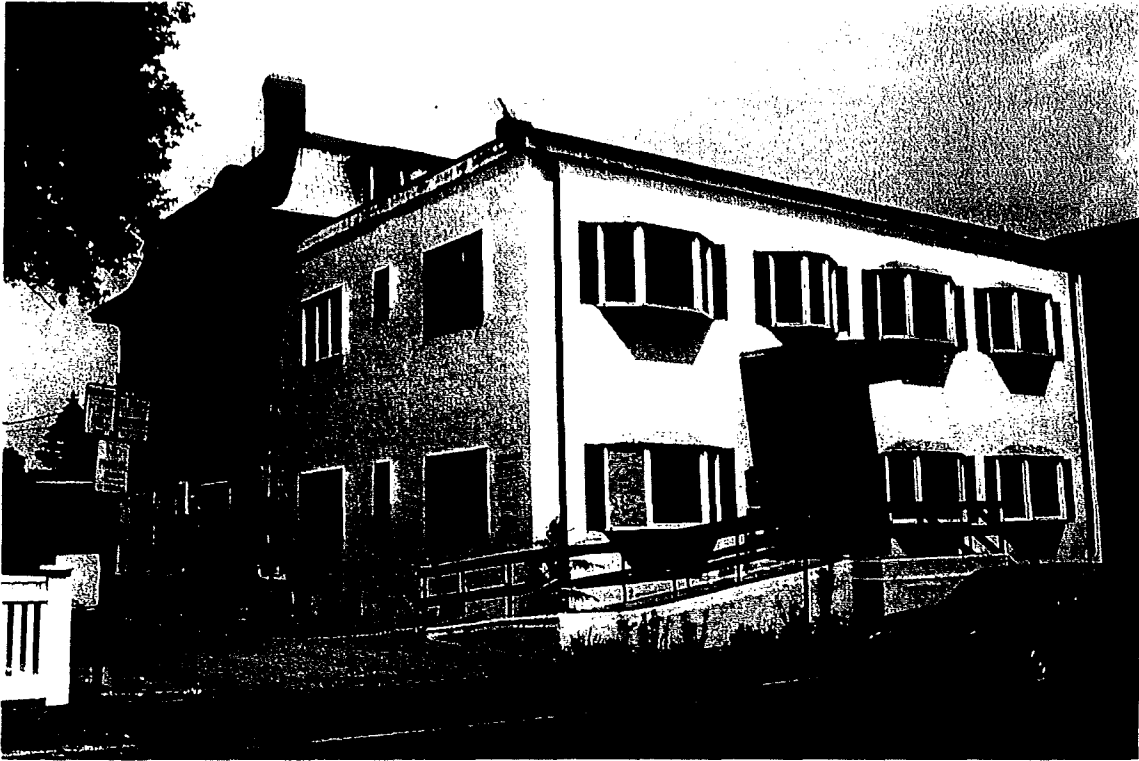
Site of Harvard Street Apartments: 273 Harvard Street, Cambridge Front - southern face of building
