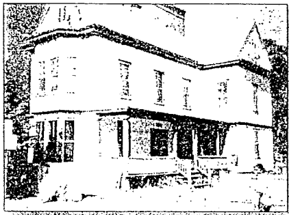
Prior to renovation
