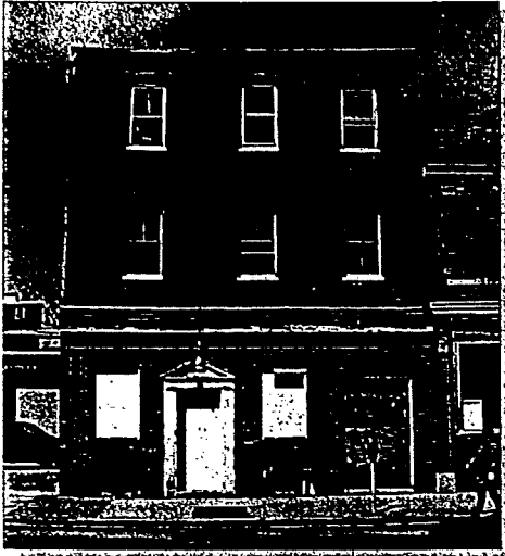
Prior to construction
