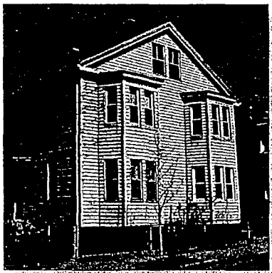
Prior to construction
