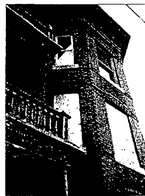
Detail of brick entrance
