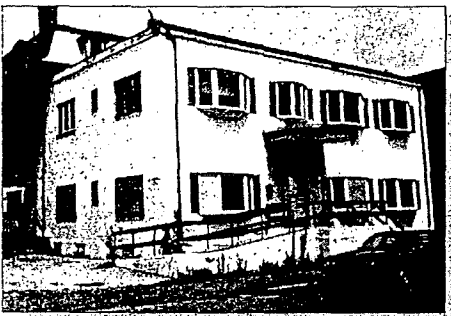
Prior to renovation
