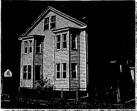
Prior to construction
