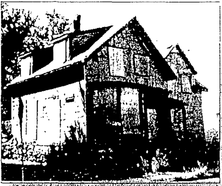
Prior to construction
