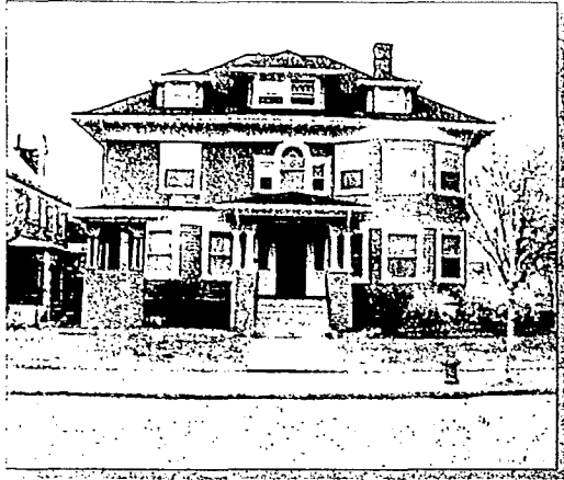
Prior to renovation
