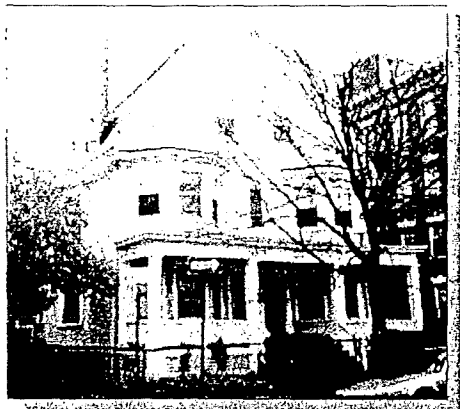
Prior to renovation
