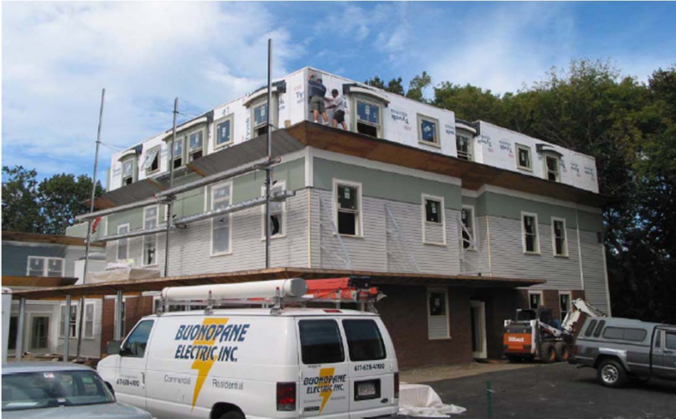
Construction as of September 2004
