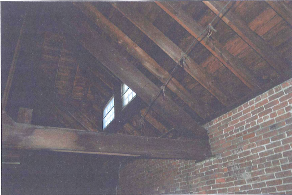
Second Floor - Wood Trusses
