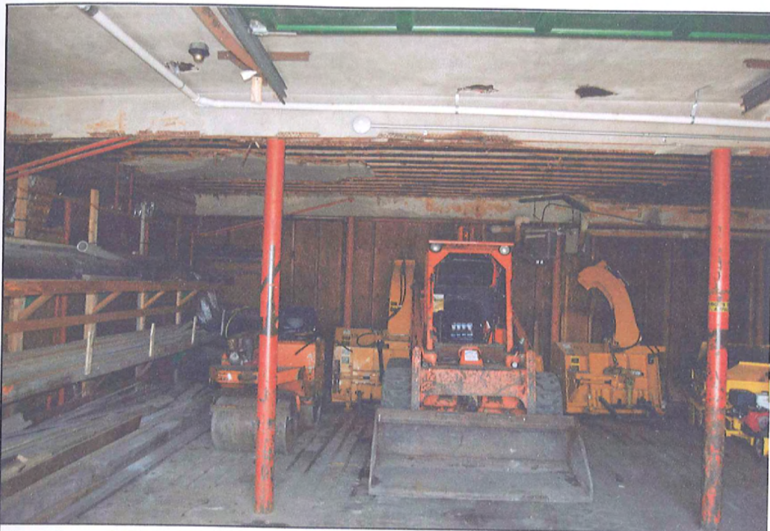
Basement - Vehicle Storage
