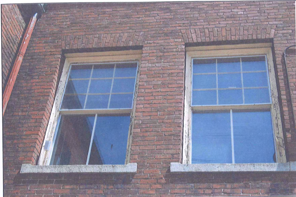
Window - First Floor - Type 4
