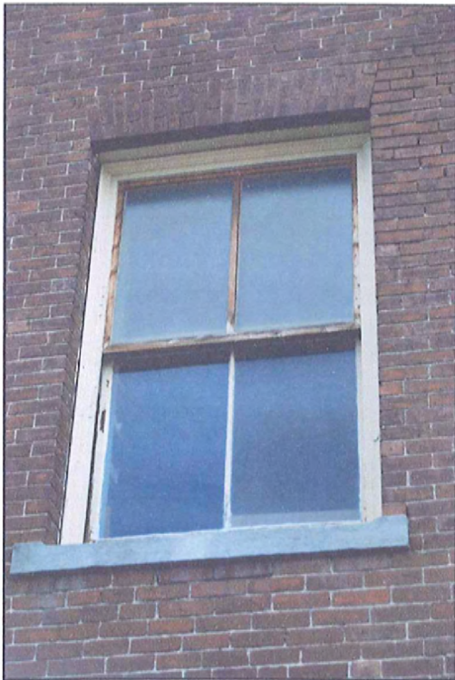
Rebuilt Window Sashes at First Floor
