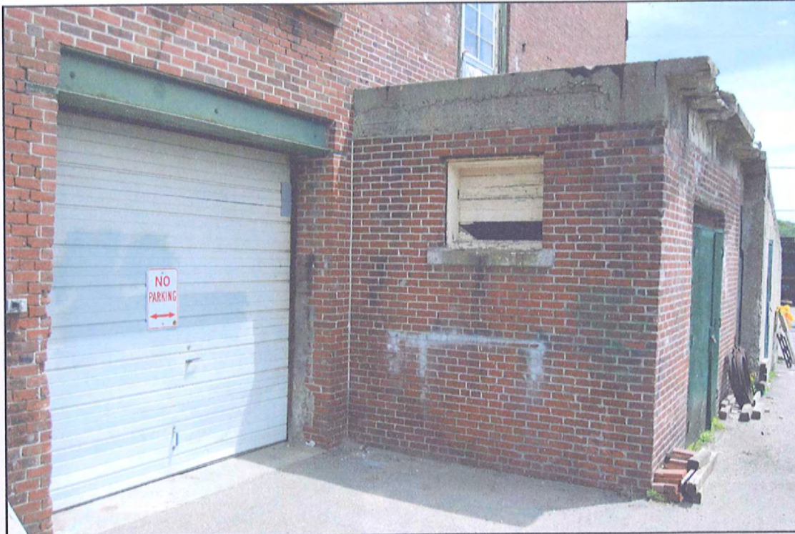
New Overhead Door - Concrete Ramp
