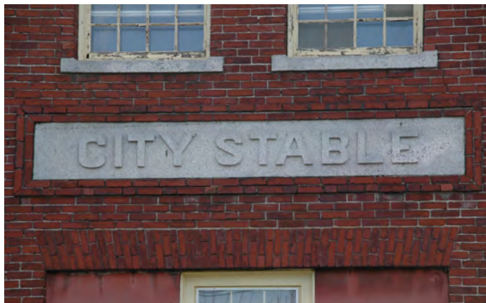
Figure 6: "City Stable" carved into a granite tablet surrounded by a brick frame
