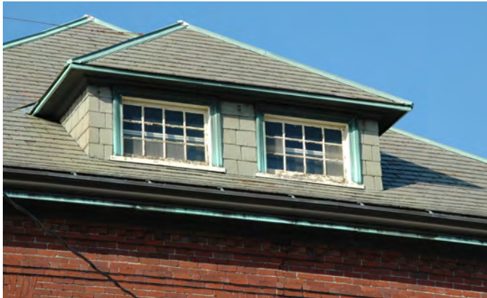
Figure 3: Typical dormer: hip roof and walls clad in slate shingles with copper flashing. Note the two 12-light wood hopper windows
