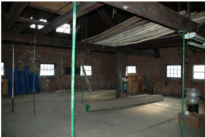
Figure 4: Attic interior. Note large platform lift set into the attic floor.
