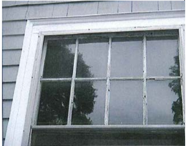
Replacement of porch windows
