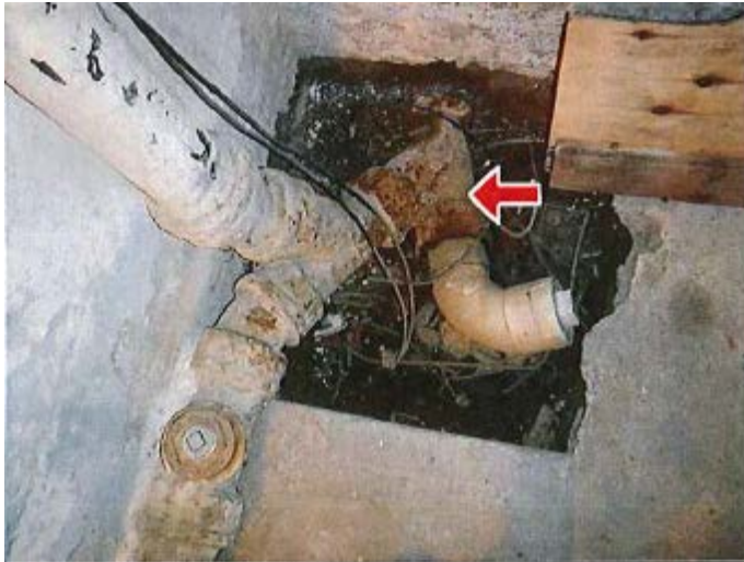
Scoping waste plumbing to determine integrity
