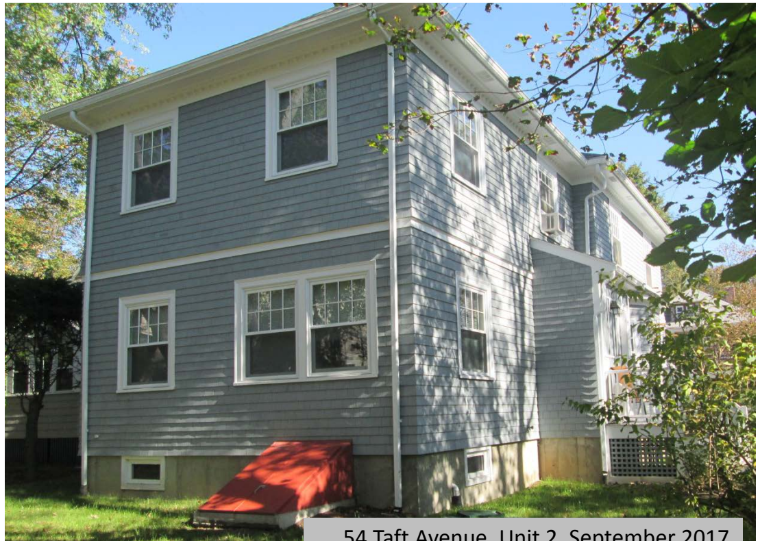
54 Taft Avenue, Unit 2, September 2017
