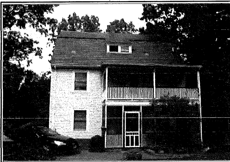
REAR OF SUBJECT PROPERTY
