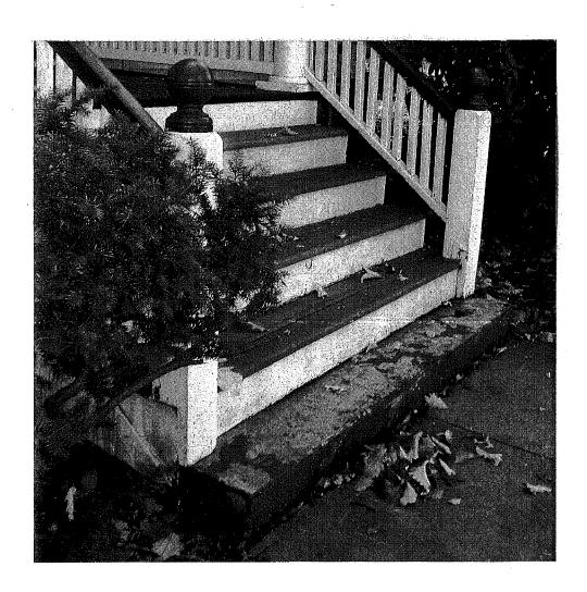
Item 3. Remove second level railings, and built-up roofing at north porch. Remove existing gutters/down spouts, and salvage same for reinstallation and install new single membrane rubber roofing, flashings and existing gutters and down spouts.
