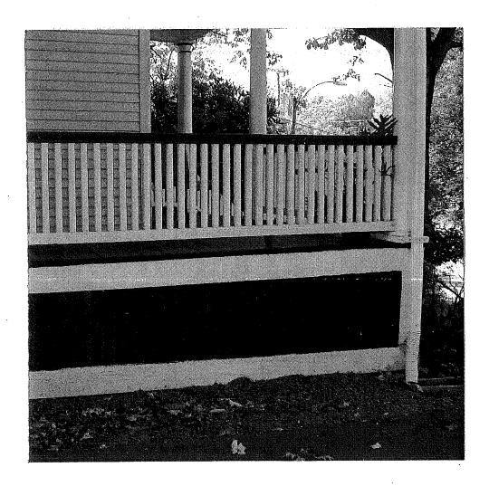
Item 11. De-lead existing exterior north and south porches newels and columns, and all interior mouthable surfaces and operable windows and doors at first and second floor units and remove and replace all vertical casings at doors and windows, where lead testing indicated positive.
