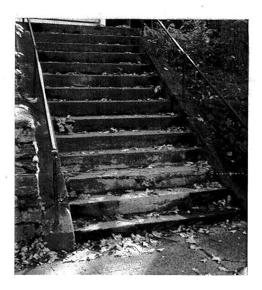
Item 2. Remove and dispose of existing concrete base and landing slab at entry upper stairs and place base material, and install new stone base and stone pavers at entry upper stairs.
