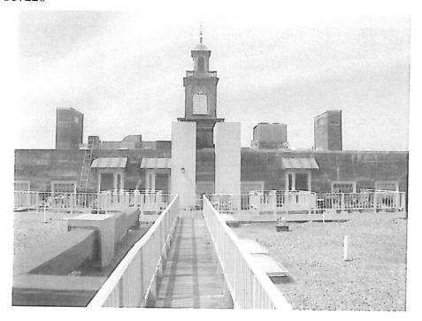
1. Overview of the various roof areas at the Warren House looking from the South Wing. Note that the low slope roof areas are typically ballasted and have wood plaza decks set atop the roof membrane.
