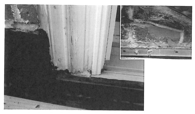
8. South Wing Roof; West Balcony. The through-wall flashings are covered with roof membrane. Brick masonry under the membrane is wet and deteriorated (refer to inset photo).
