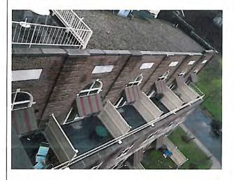
Southwest balcony roof: Existing railing systems did not comply with spacing of balusters per the Massachusetts State Building Code (MSBC). Severe water infiltration was reported at the apartment units below the balconies. Cast stone copings are uncovered with multiple areas of cracked and spalled stone.
