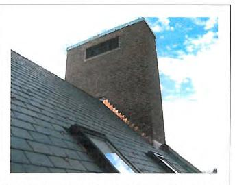
The chimneys that were included in the Phase I scope were repointed, louvers were refurbished to incorporate proper head and sill flashings, throughwall flashings at the base of the chimneys were replaced to address the water infiltration.
