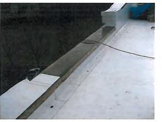
Cast stone parapet stones were flashed over with the thermoplastic roofing membrane and capped with copper. Areas of missing stone were filled in with wood blocking to minimize costs of replicating cast stone that would be covered with copper.
