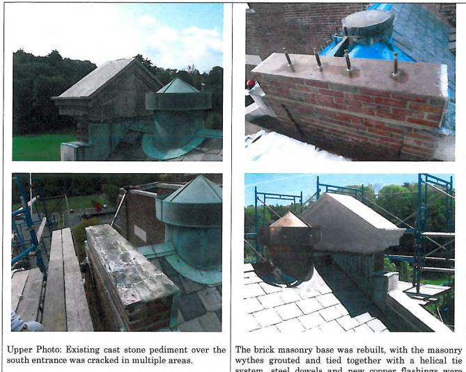
Lower Photo: Removal of the pediment revealed that there were no supporting steel elements through the masonry below, and it was set on the flashing in the lower photo. Upon removal of the stone, the brick masonry base was unstable and required rebuilding.
