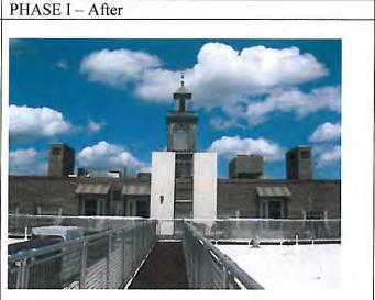
View from the south roof stairwell looking north: new thermoplastic roof systems with tapered insulation and overflow drainage accommodations, new railings, walkway and deck systems. Masonry repairs and 100% repointing was performed at all the above roof line components within the Contract limits.
