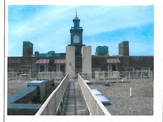
View from the south roof stairwell looking north: ballasted EPDM roofs installed circa 1993 were at the end of their service life with multi areas of ponding and poor drainage. Multiple leaks were reported at the penthouse units. Existing railing systems did not comply with spacing of balusters per the Massachusetts State Building Code (MSBC).
