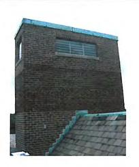
Multiple leaks were reported at the apartments adjacent to the chimney walls. Plexi glass had been installed over the louvers as a temporary waterproofing measure. Spot repointing of the chimneys and sealant and mastic repairs on the adjacent copper flashing and slate roof areas were performed.
