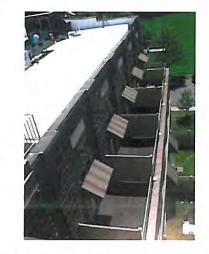
Southwest balcony roof: Refurbished railing systems, new balcony waterproofing systems, new throughwall flashing systems, copper caps over all the existing cast stone copings, repainted wood balcony and transoms including wood repairs of rotted wood components.
