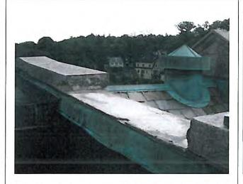
Several cast stone parapet stones were identified in 2009 as being potential fall hazards and removed until renovation work could be performed.
